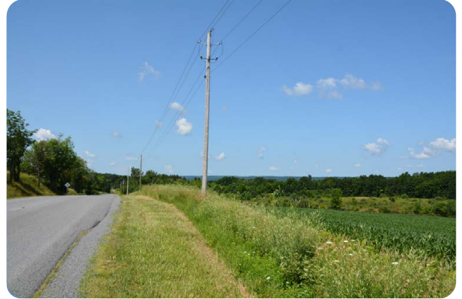
Example of existing roadside vegetation (Dutch Street Road).
