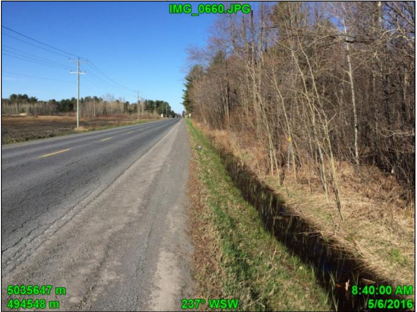
Station 1: Facing upstream (west), north side of road.
