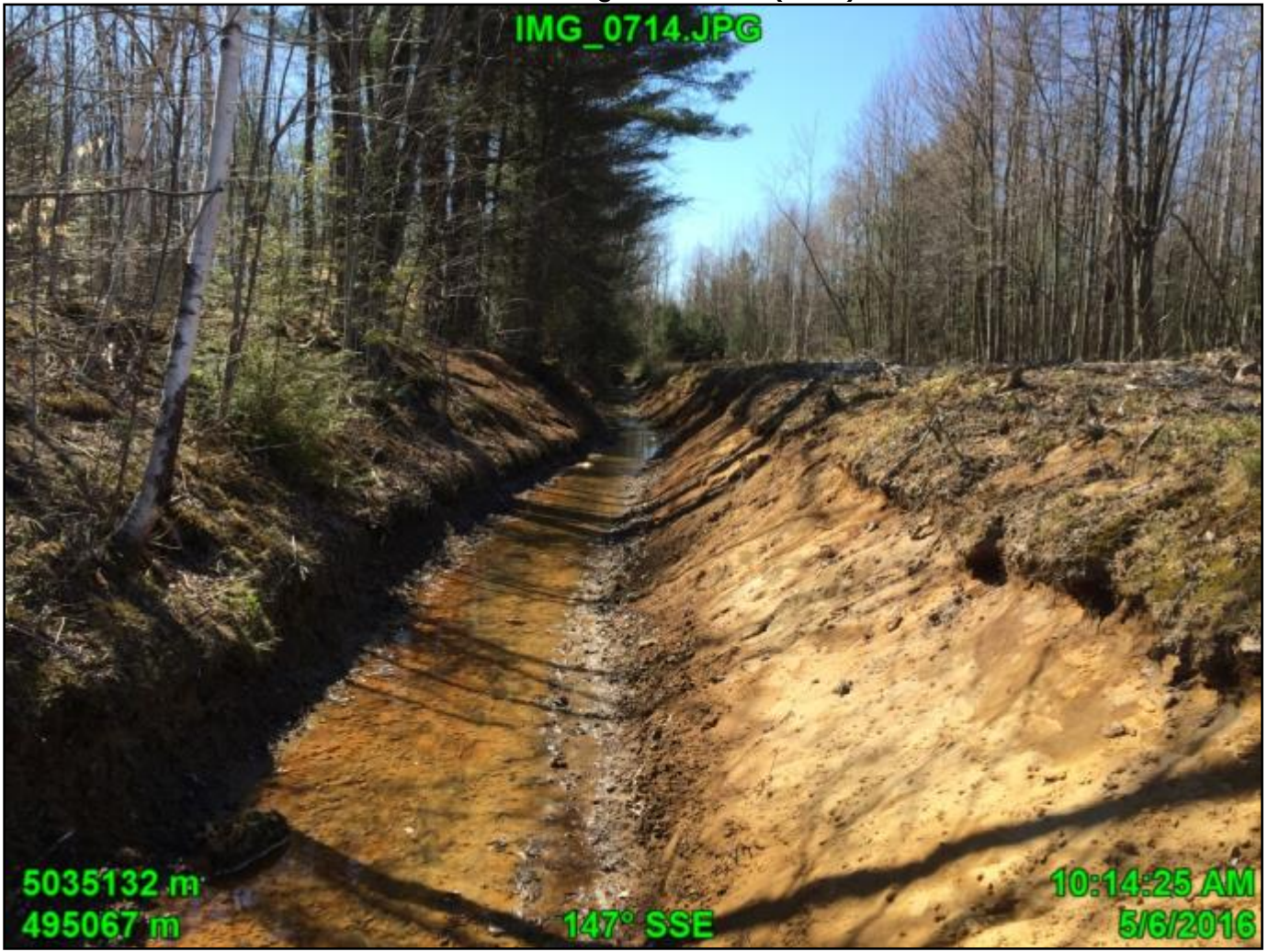
Station 4: F facing downstream (south).
