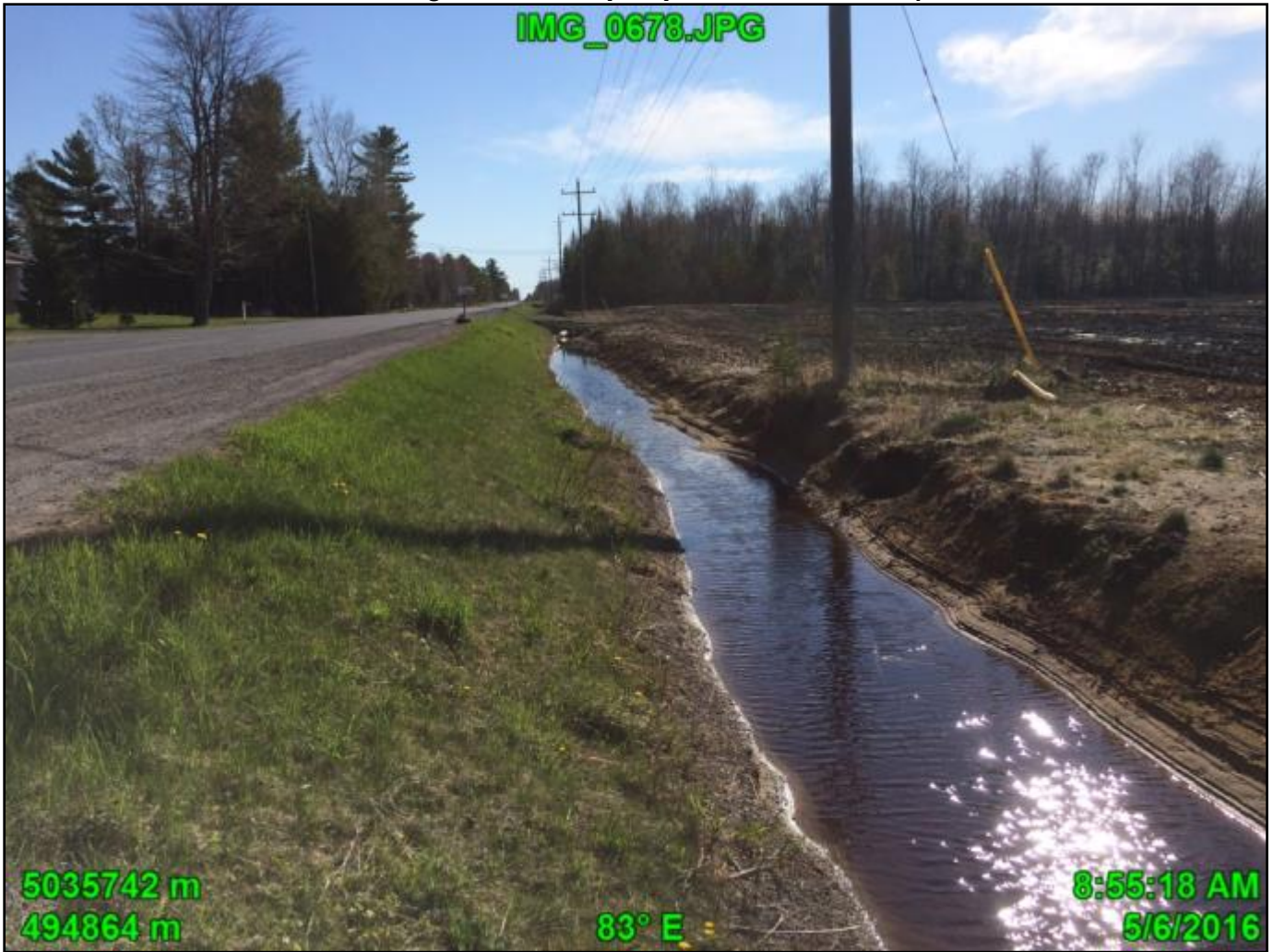
Station 1: Facing downstream (east), south side of County Road 2.
