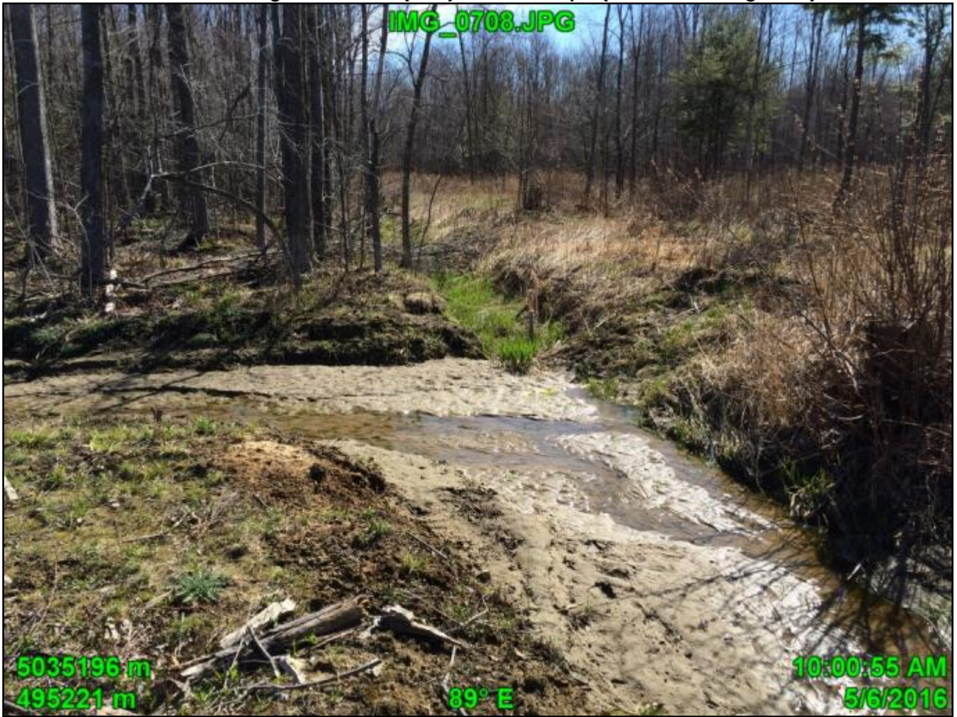
Station 6: Facing downstream (east) at channel split (Station 3 in foreground).
