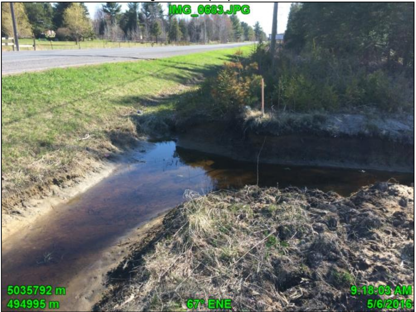
Station 1: Facing downstream (east) at east end of Station 1.
