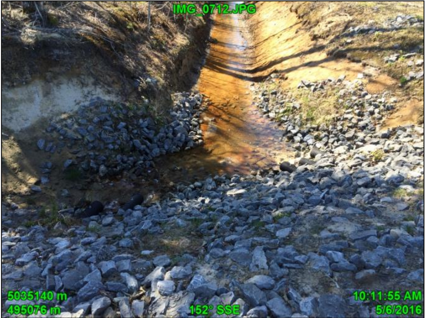
Station 4: Facing downstream (south) from tile outlet near south edge of property.
