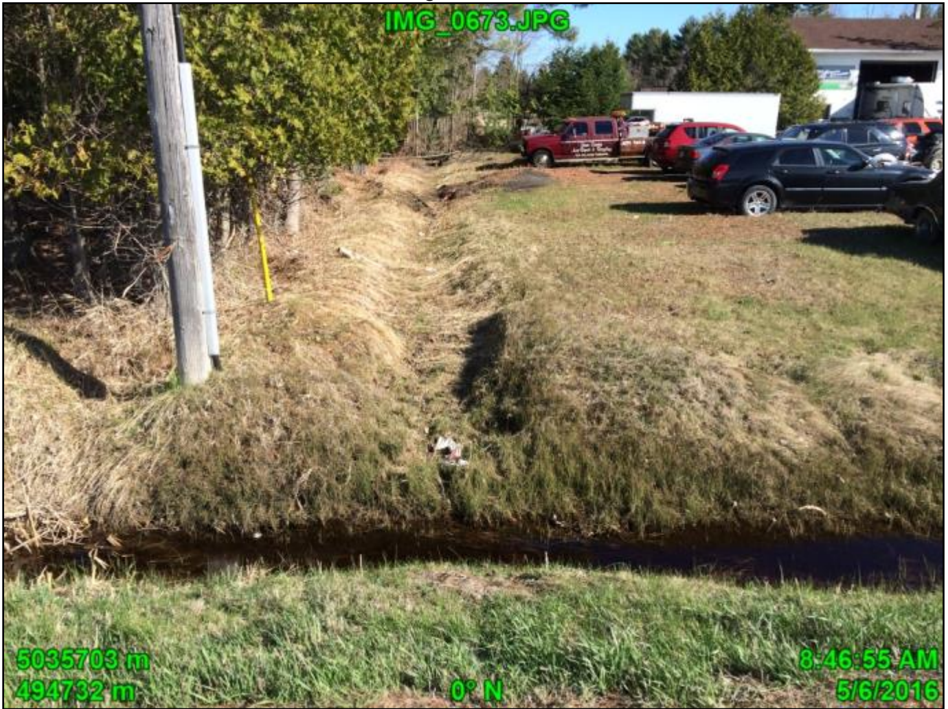
Station 1: Facing north, north side of road.
