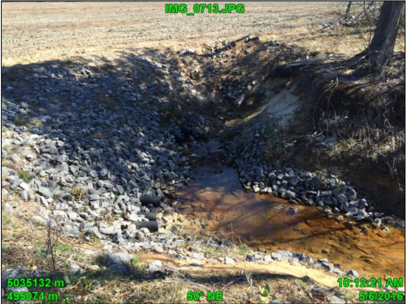
Station 4: Facing north toward tile outlet at south side of the project.
