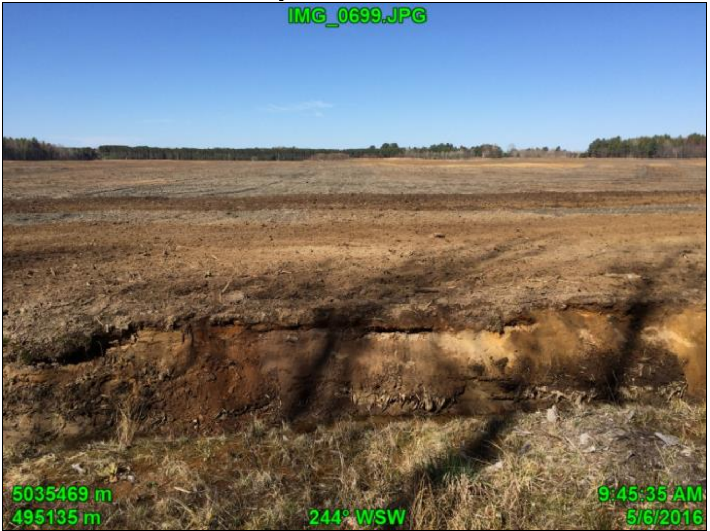
Station 2: Facing southwest from east side of Station 2.
