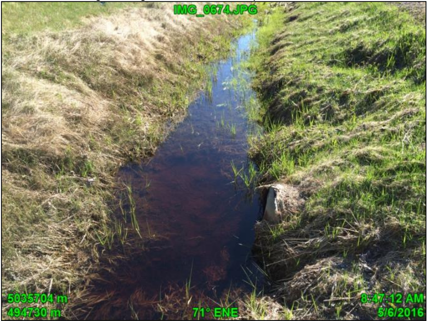
Station 1: Facing east along roadside ditch from County Road 2 culvert, north side of road.
