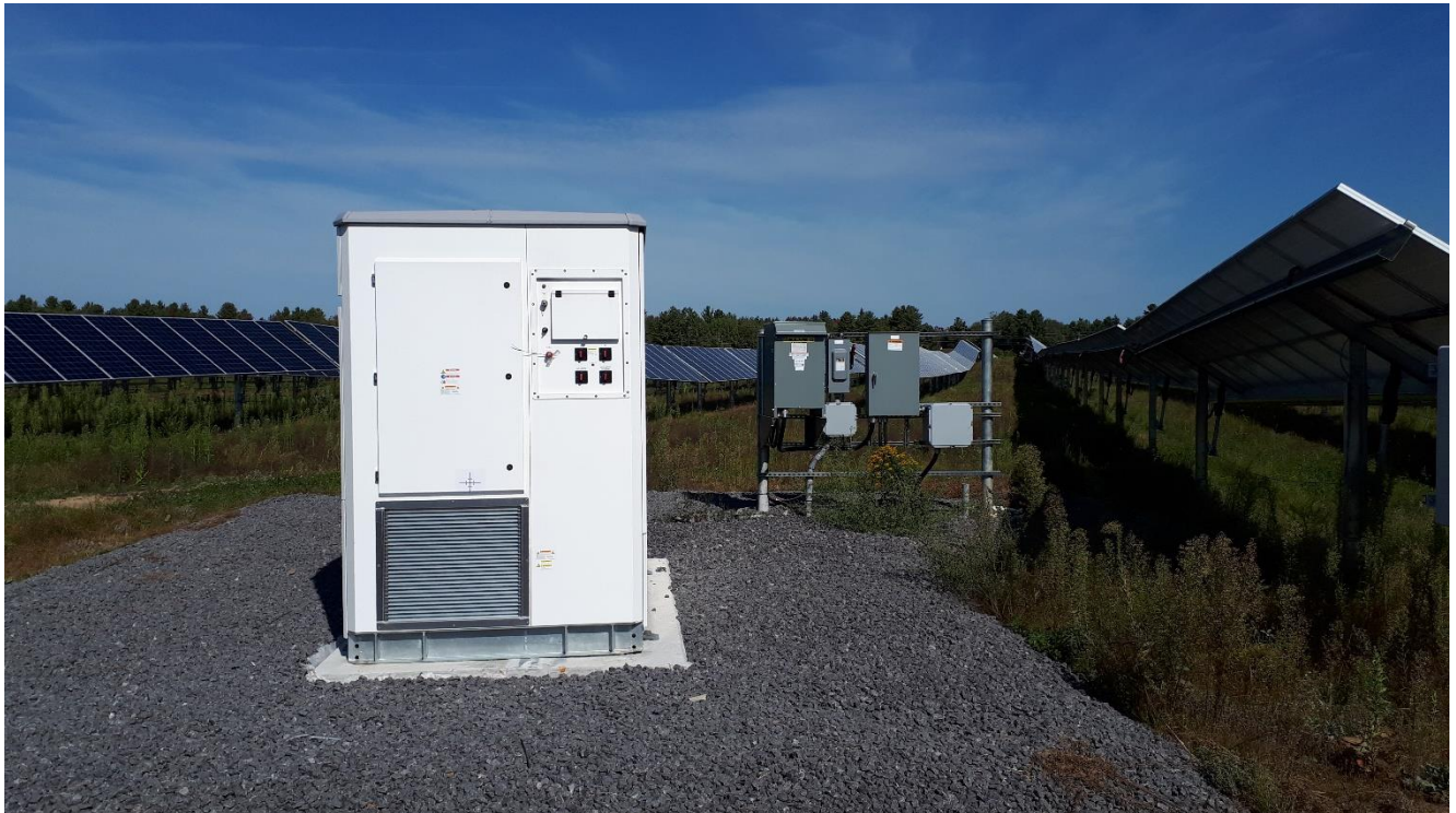
Figure A-4 Inverter cluster 4
