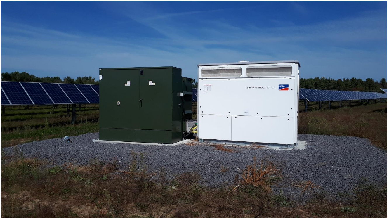
Figure A-3 Inverter cluster 3
