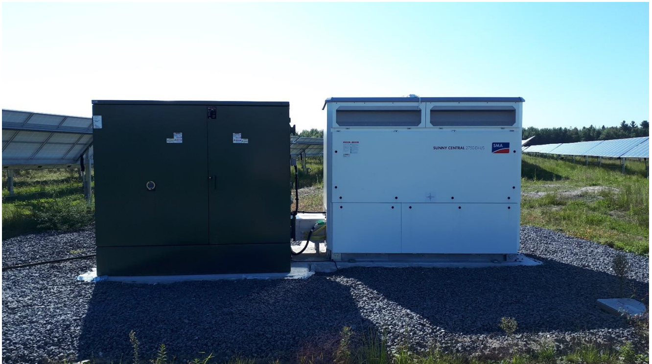
Figure A-2 Transformer / Inverter Cluster 2
