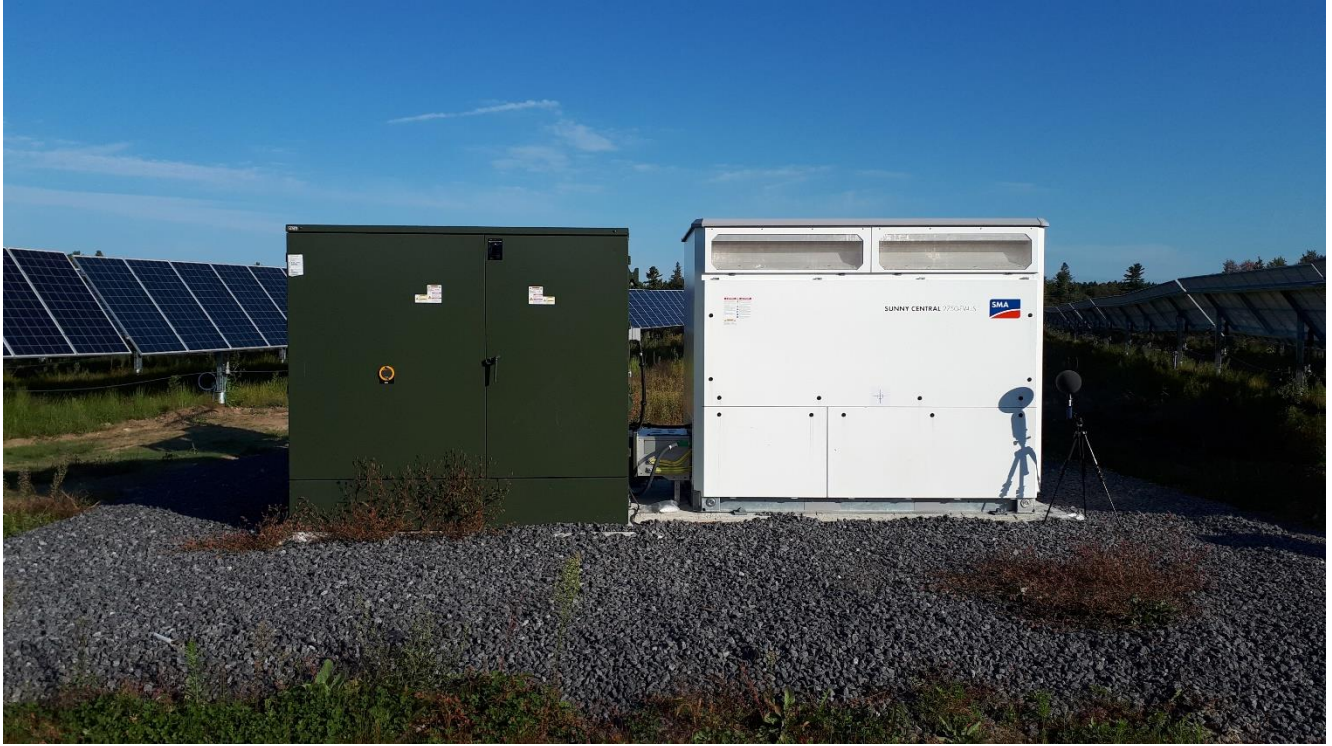
Figure A-5 Inverter cluster 5
