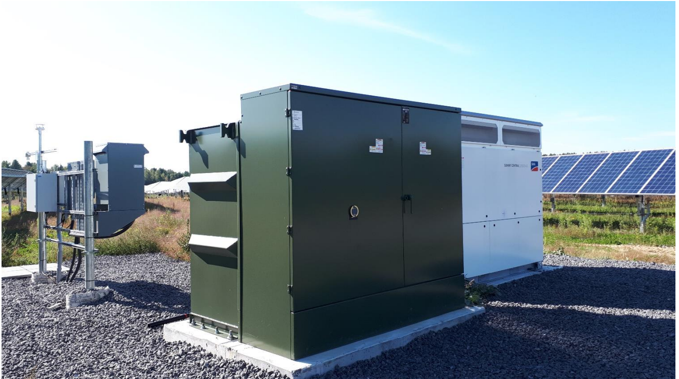
Figure A-1 Transformer / Inverter Cluster 1
