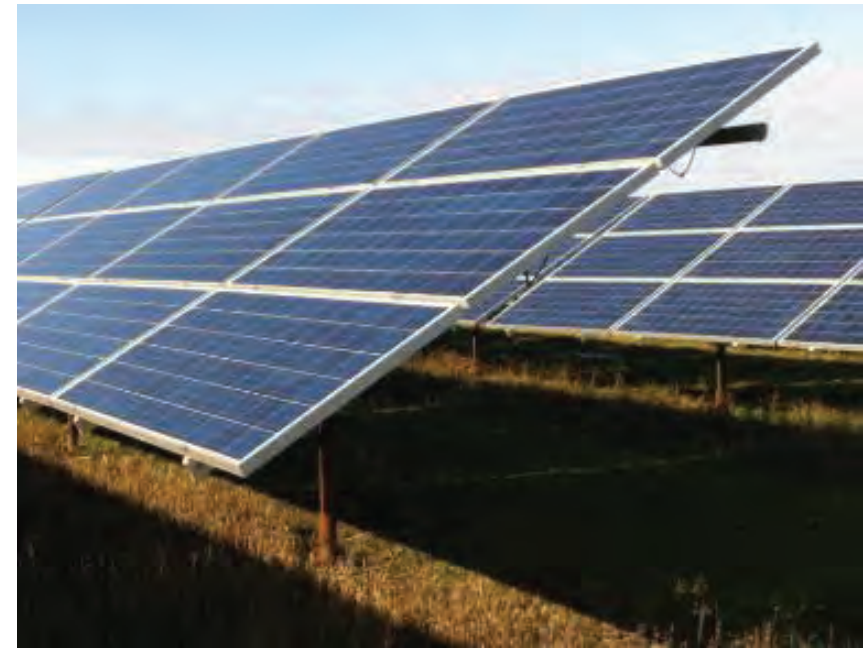
Fixed tilt – bottom of panel > 30 cm above floodplain level
