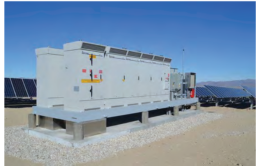
Sample Inverter/Transformer Skids
