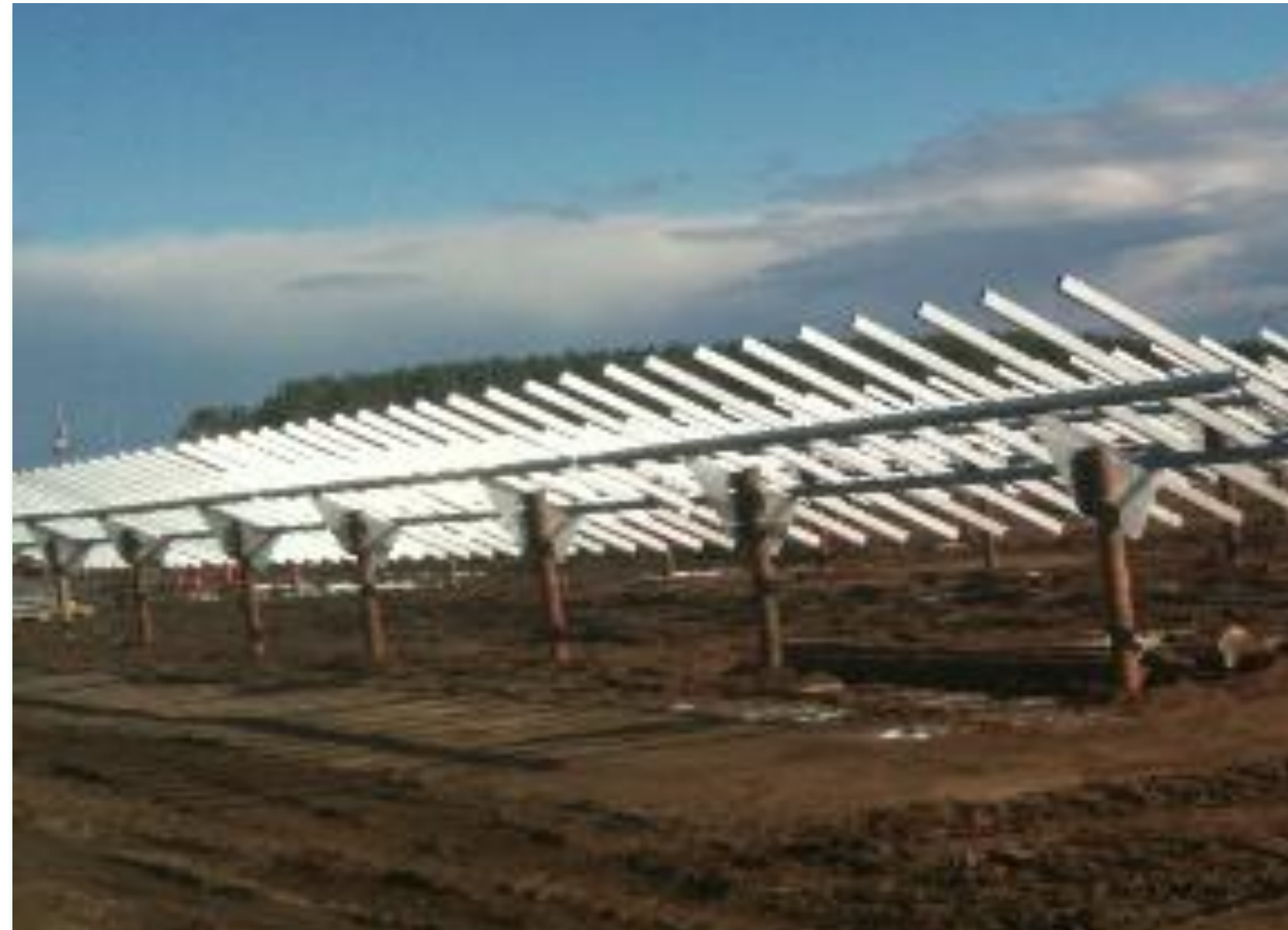
Install Piles and Racking
