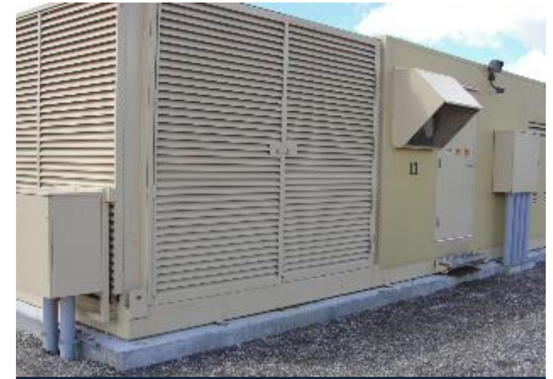
A few inverters/transformers condition power to be compatible on local electricity grid
