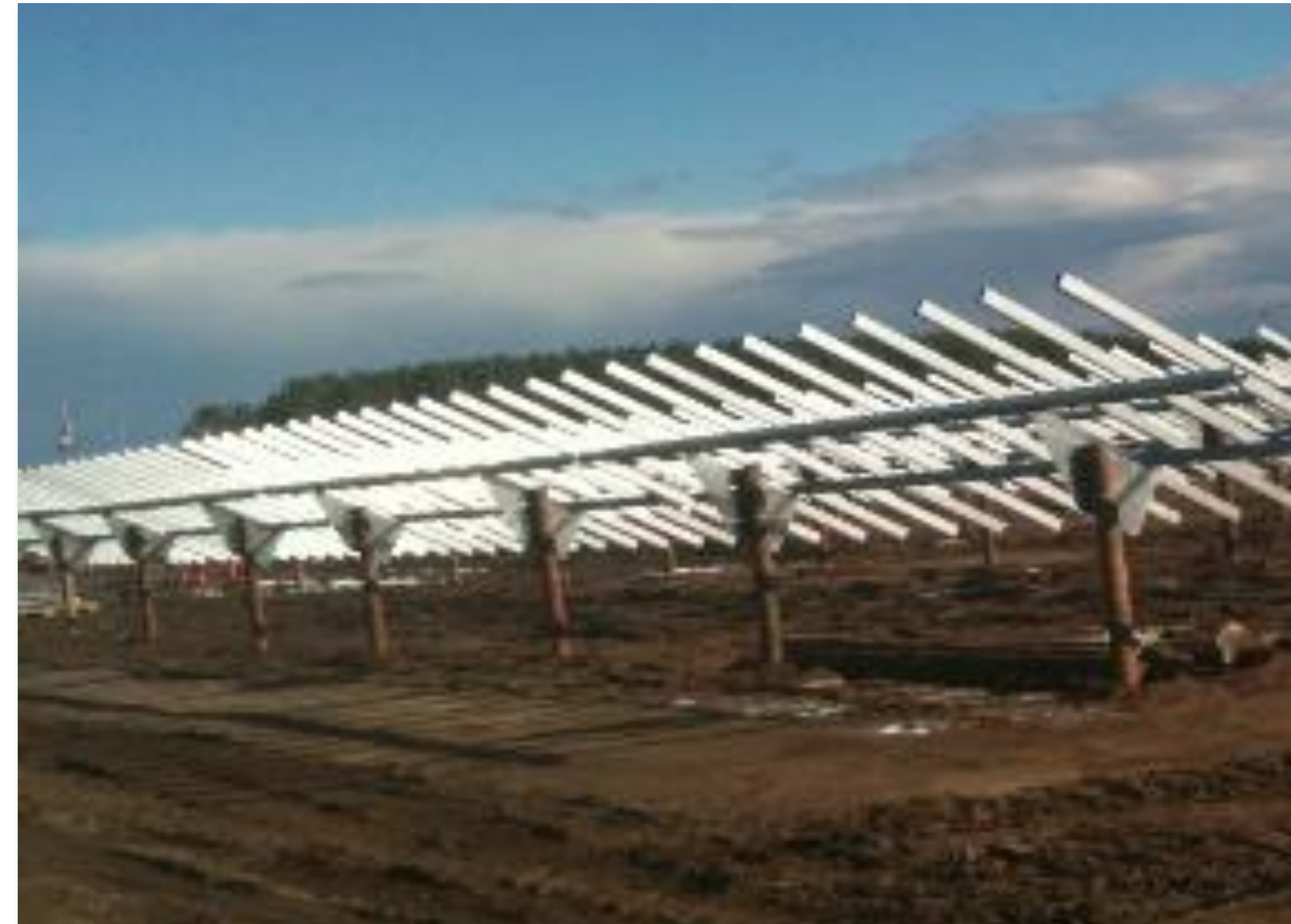
Install Piles and Racking
