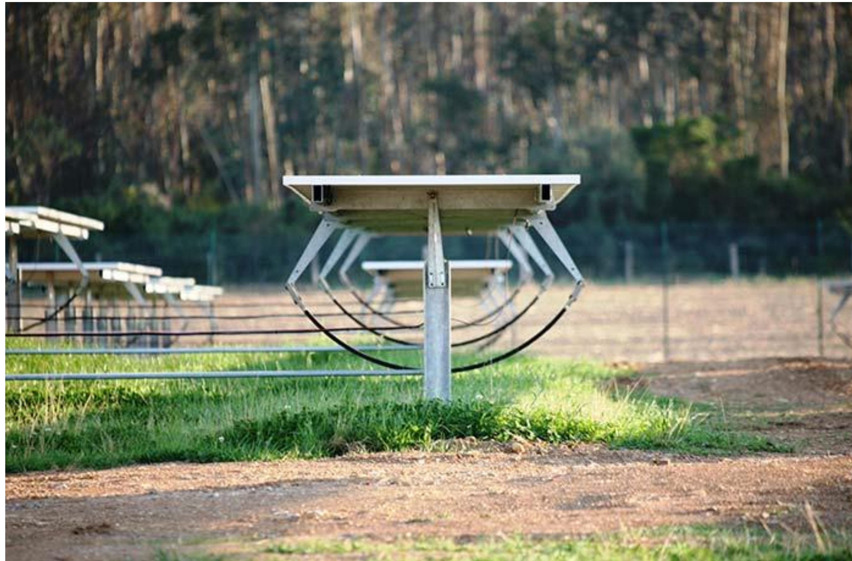
Solar Panels Mounted on Tracker System Panels Track the Sun from East to West Source: http://www.exosun.net/references/photo-gallery
