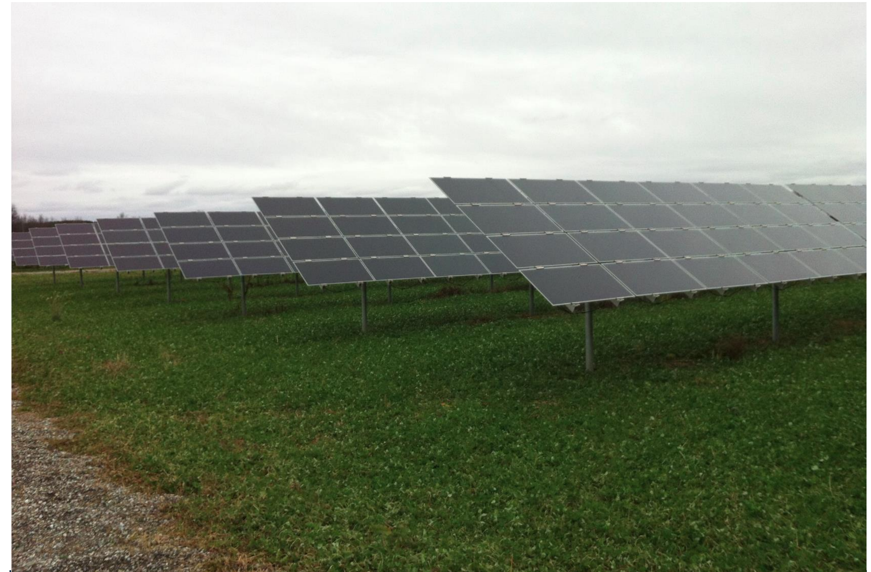
Fixed Tilt System Solar Panels do not Move
