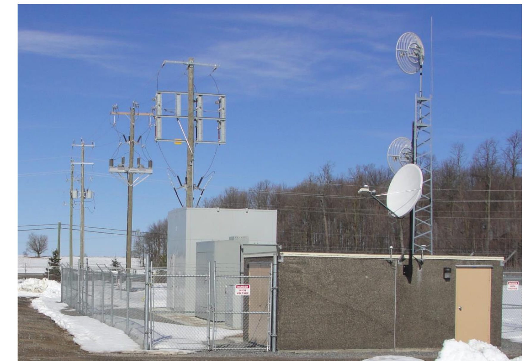
Substation includes necessary equipment to connect to the local electricity grid
