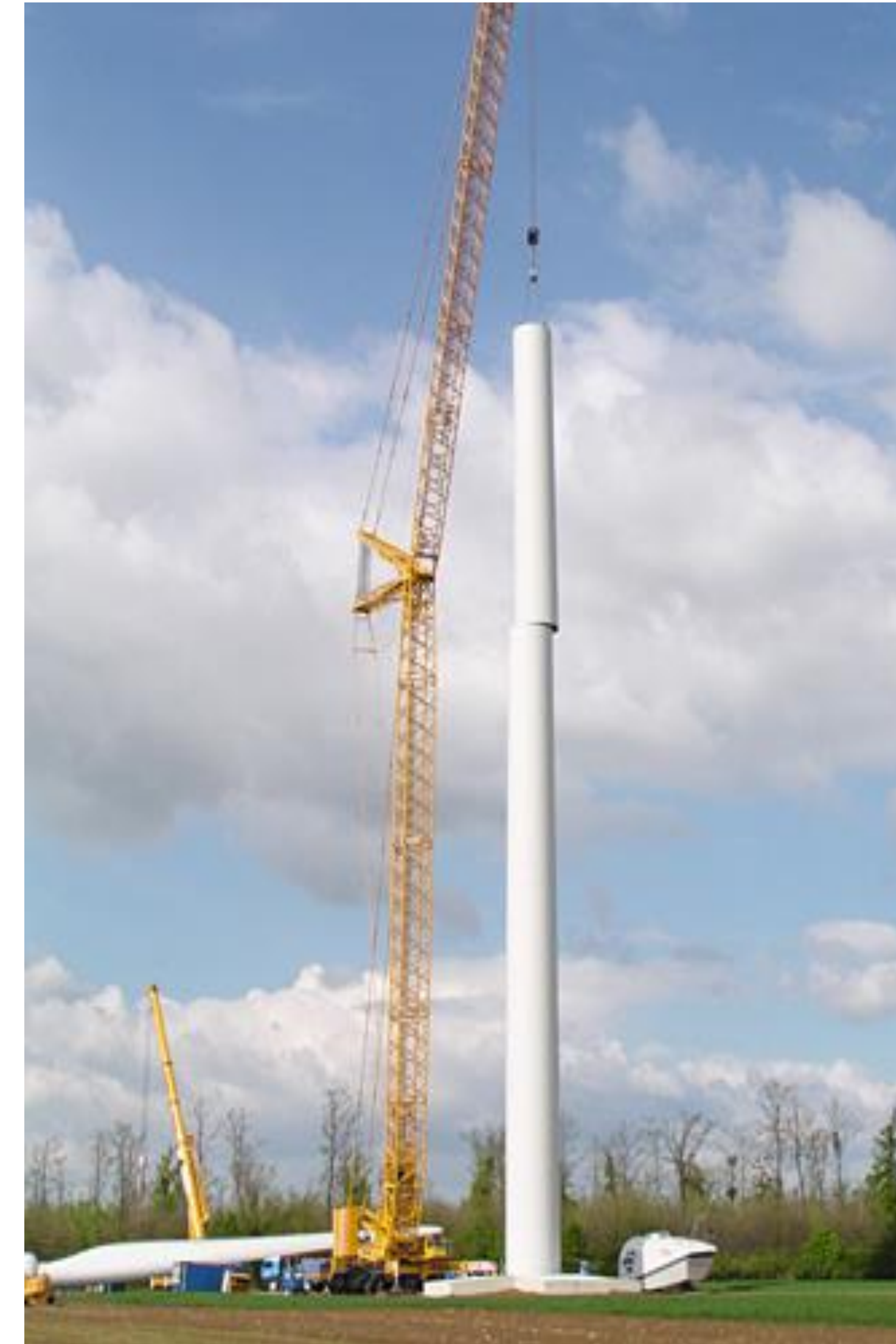
Nacelle installation The nacelle weighs about 65 tons.
