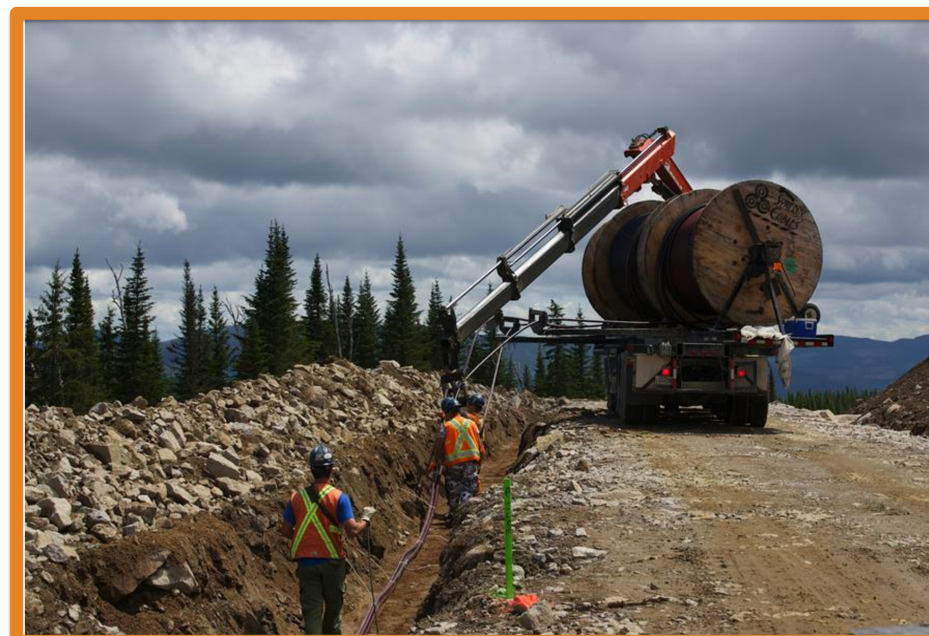
Buried collection system
