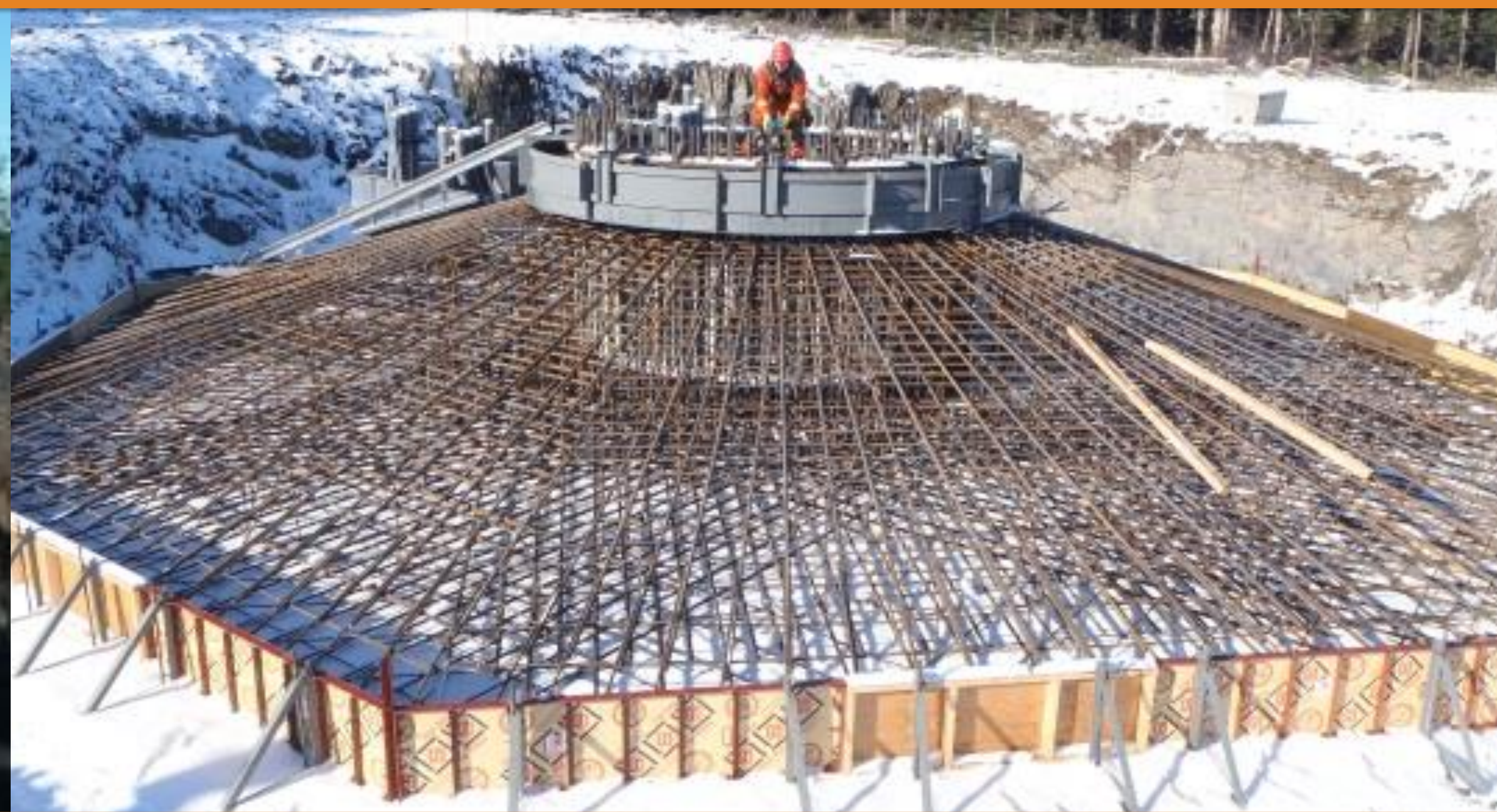
Reinforcing steel installation. Between 40-50 tons of rebar
