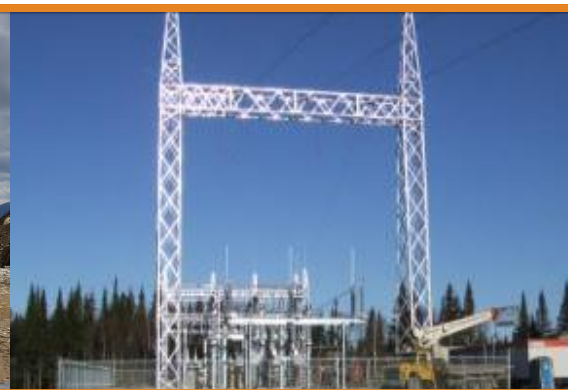
Substation connecting the project to the Hydro One 230 kV transmission line
