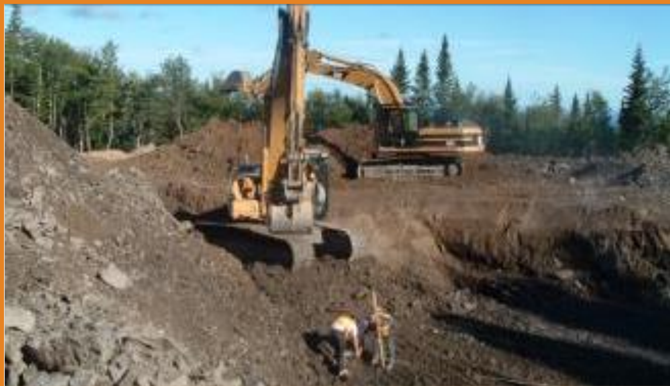
Foundation excavation. Diameter approx. 20 m
