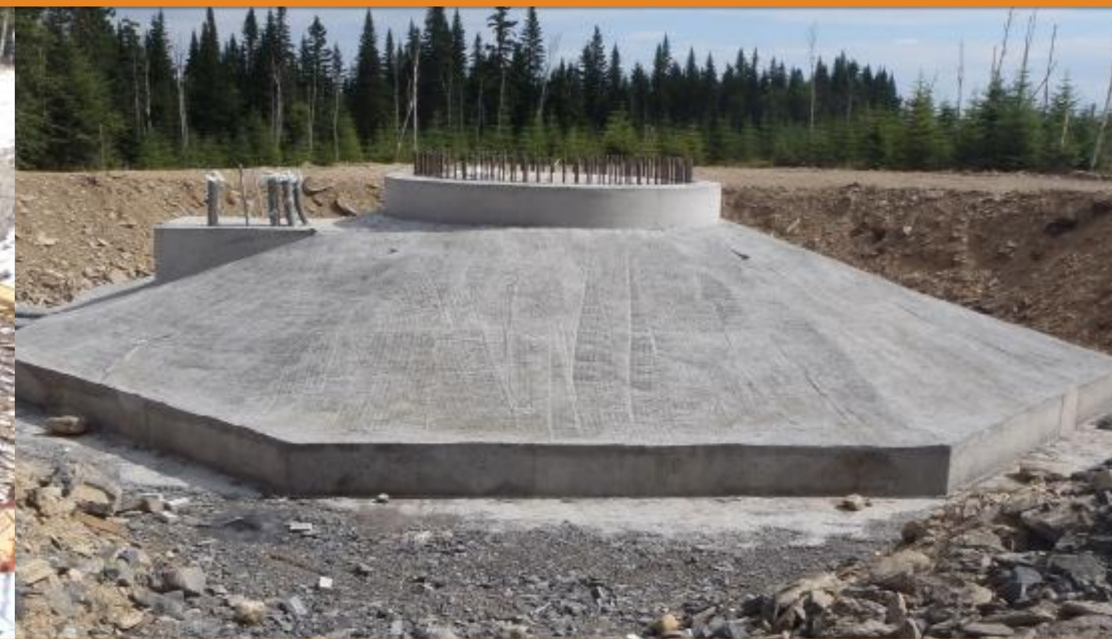
Concrete pouring. Approx. 400-600 m 3 of concrete per foundation
