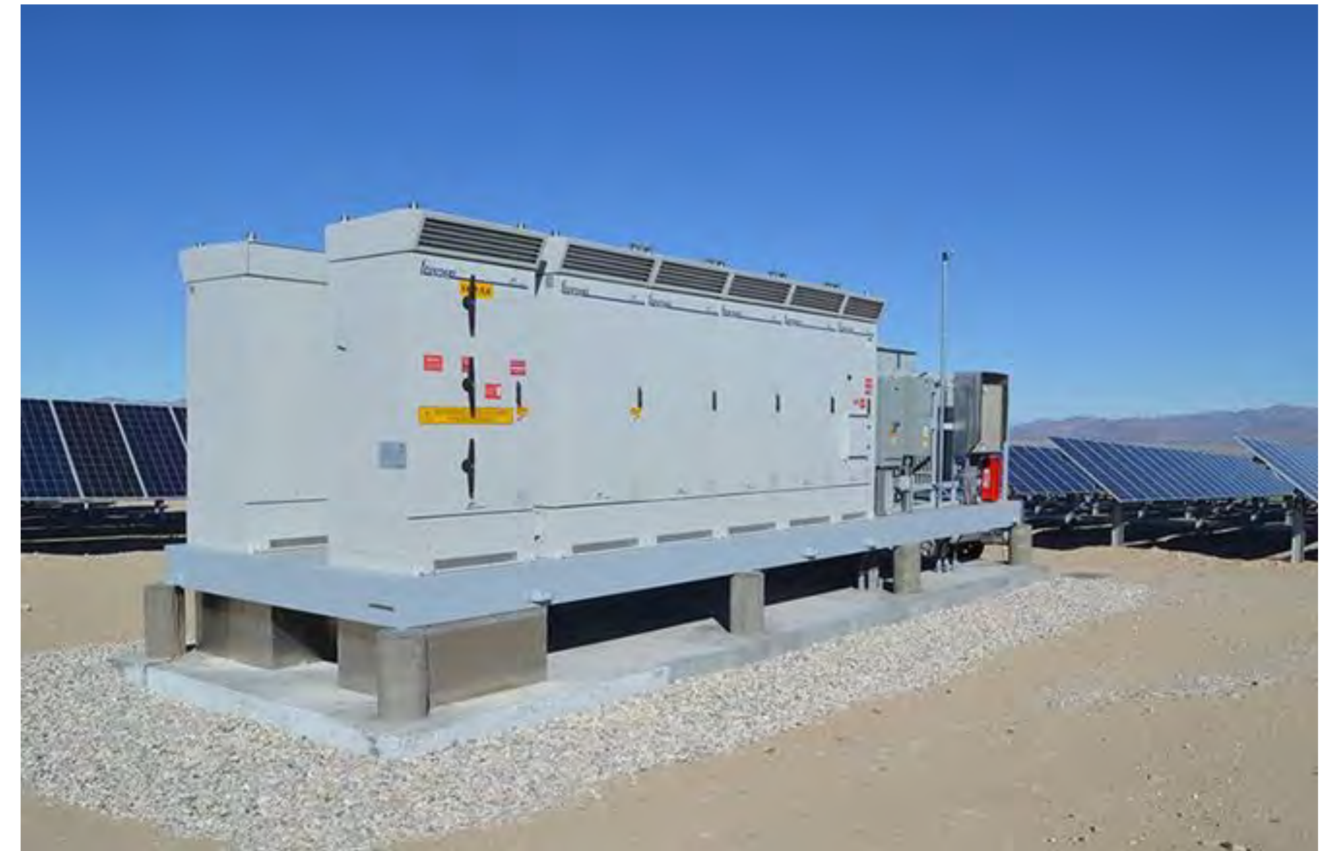
Sample Inverter/Transformer Skids
