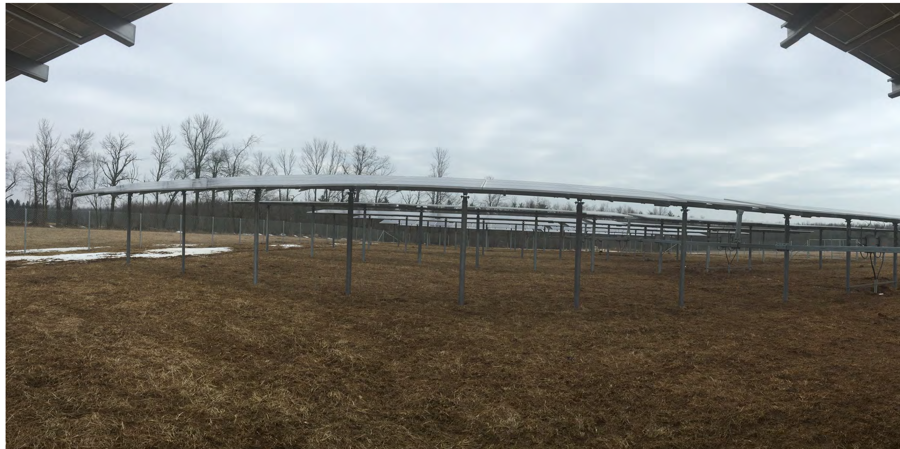
Example of Horizontal Single Axis Tracker in Table Position
