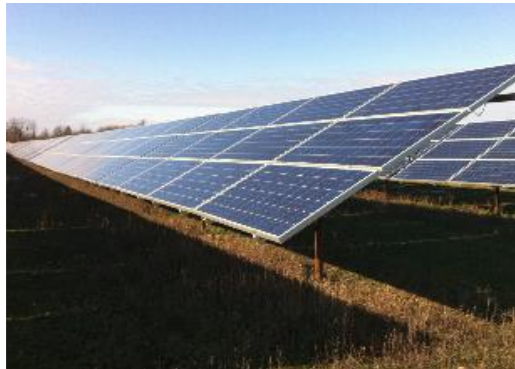
Finished Product (view from ground)
