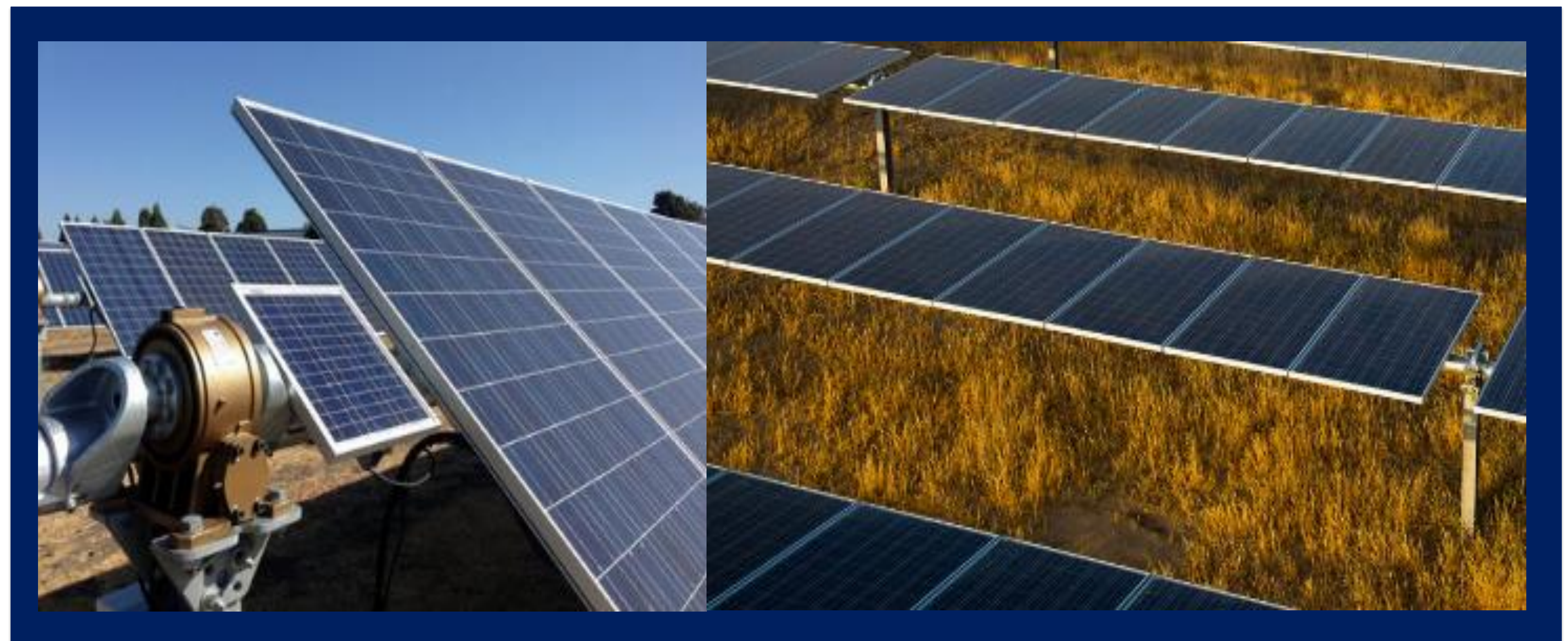
Horizontal single axis tracking
