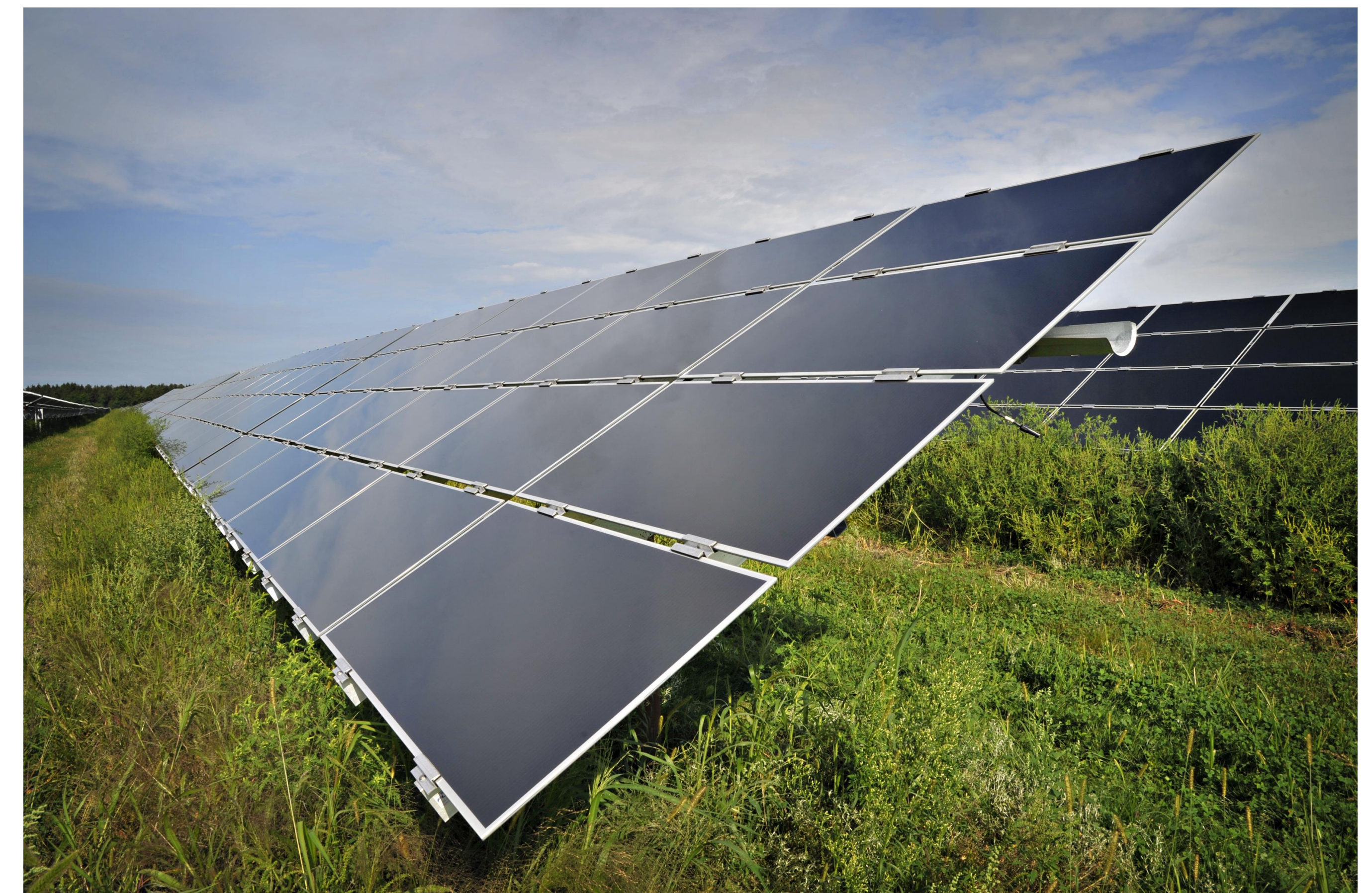
Vegetation around / beneath panels
