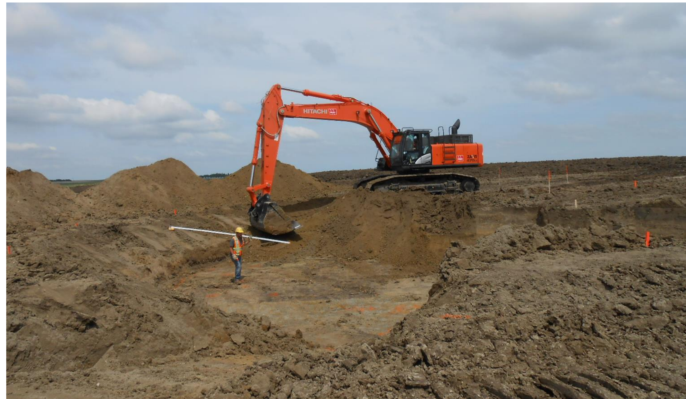
Foundation excavation. (Diameter approx. 20 metres)
