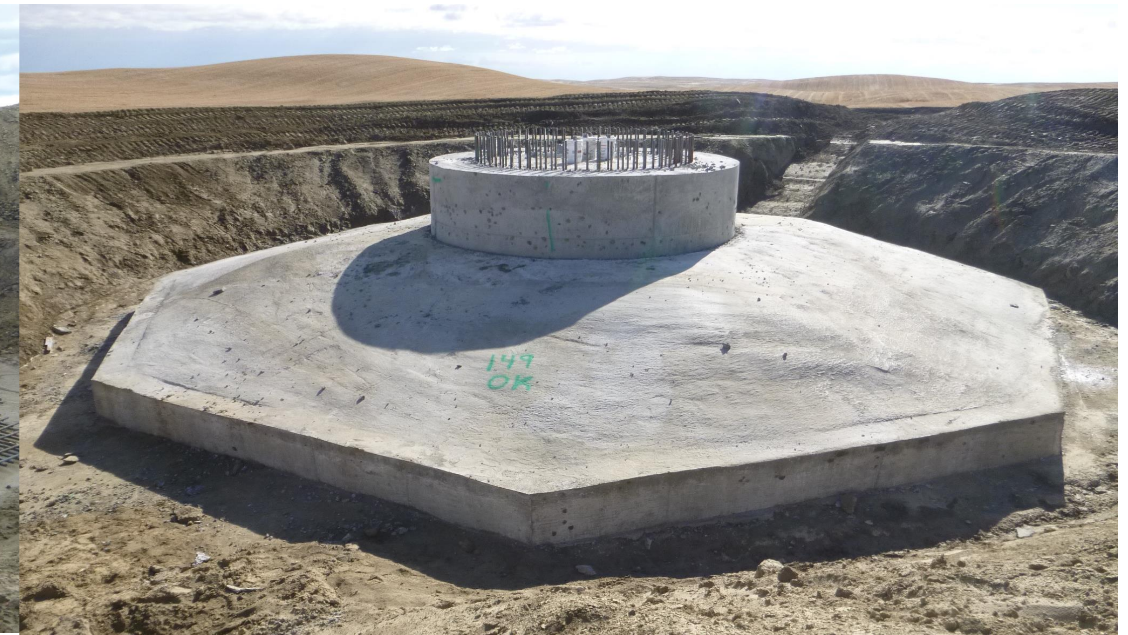
Each foundation requires approx. 400-600 m3 of concrete.
