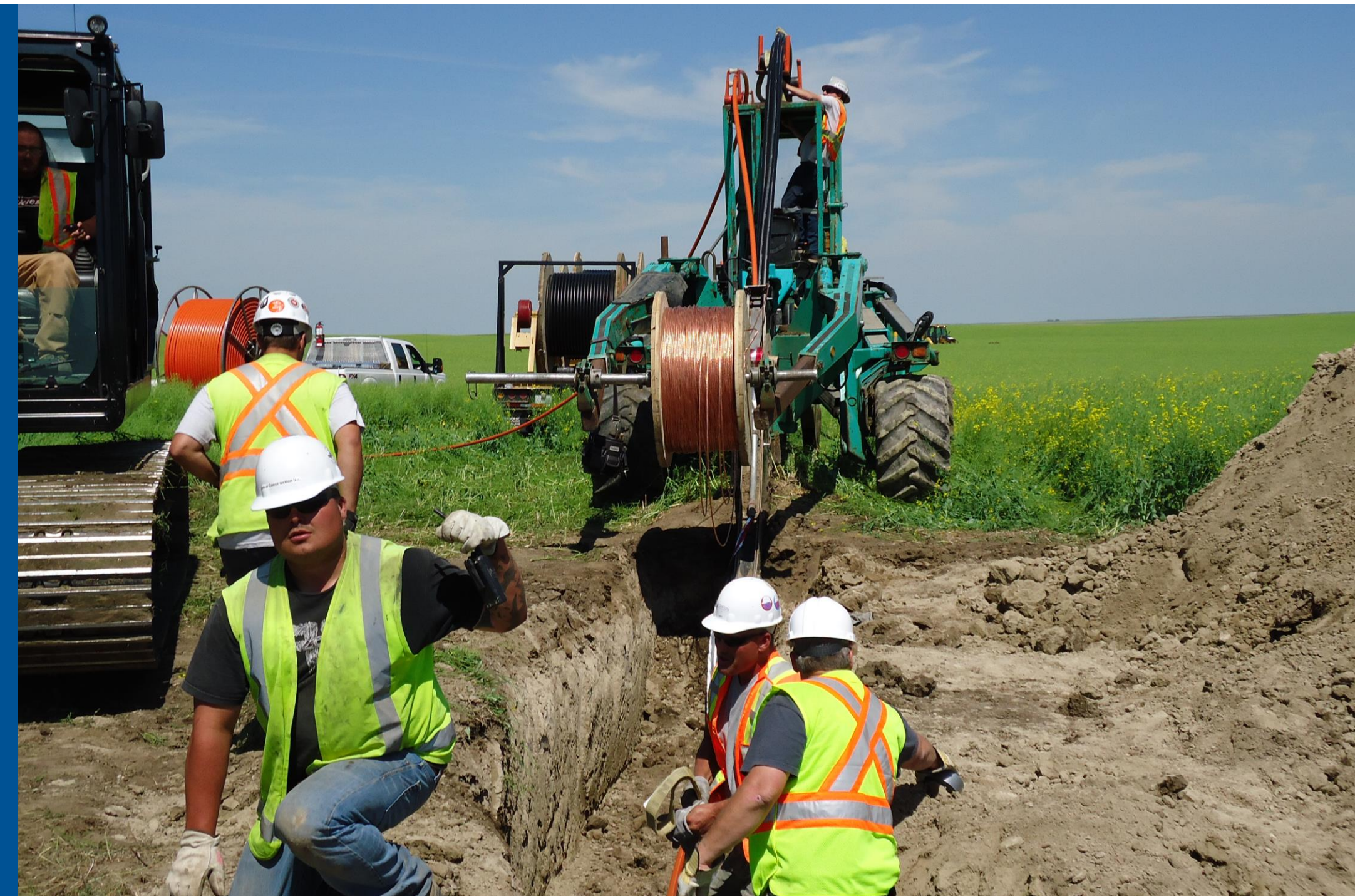
Buried collection system
