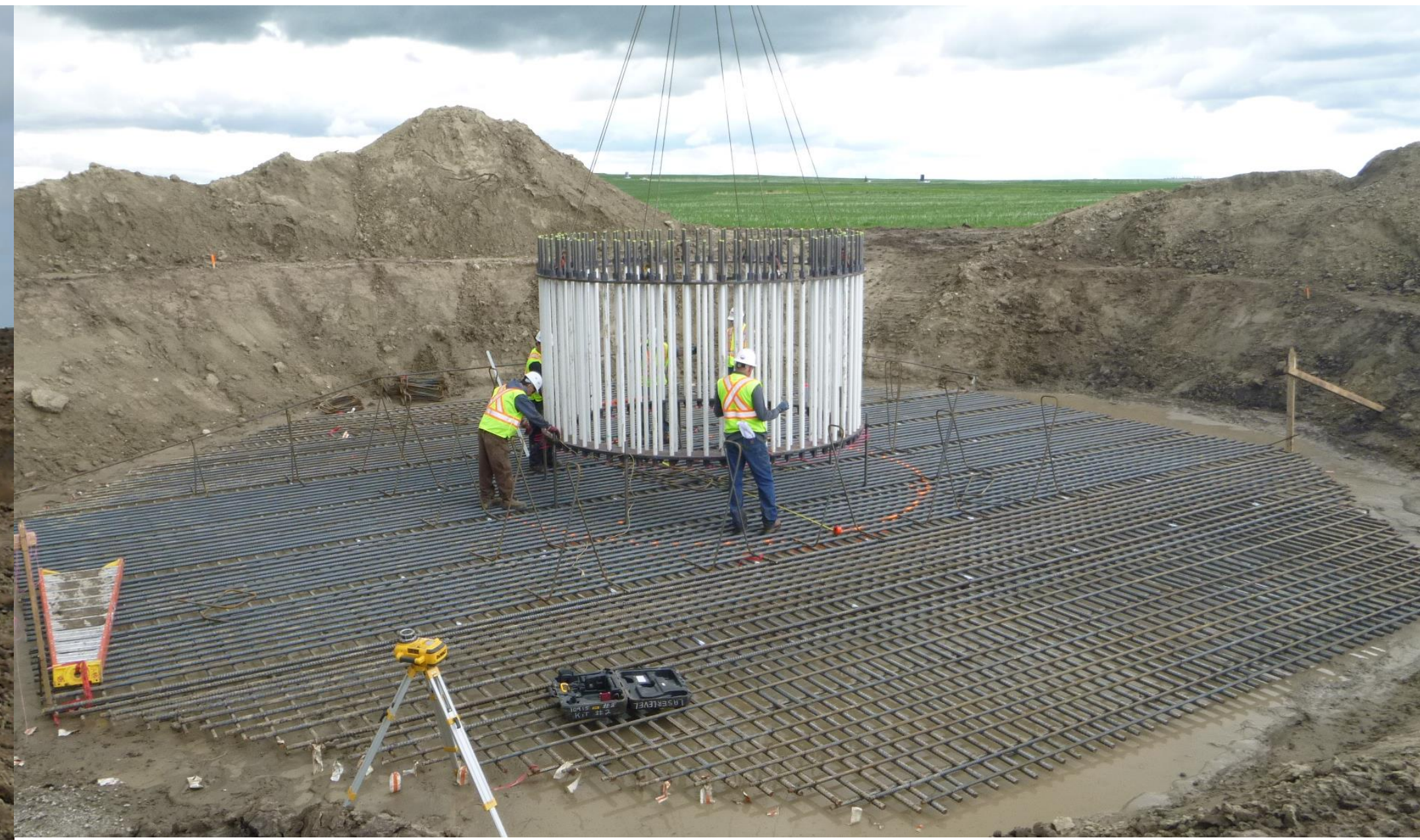
Reinforcing steel installation. Between 40-50 tons of rebar.
