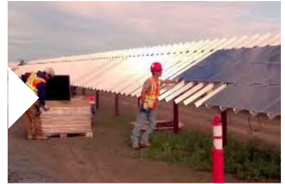
Panels installed on racking
