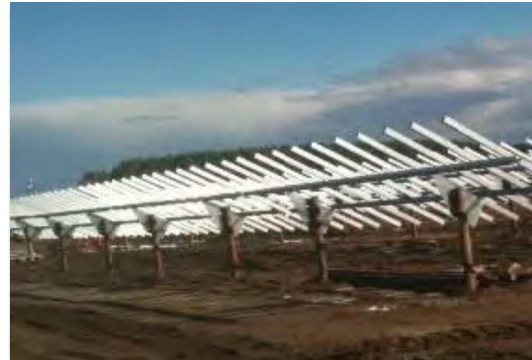
Racking mounted on piles
