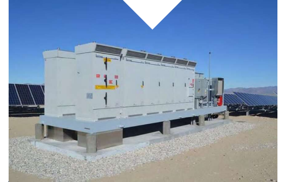
Inverter/Transformer Skid
