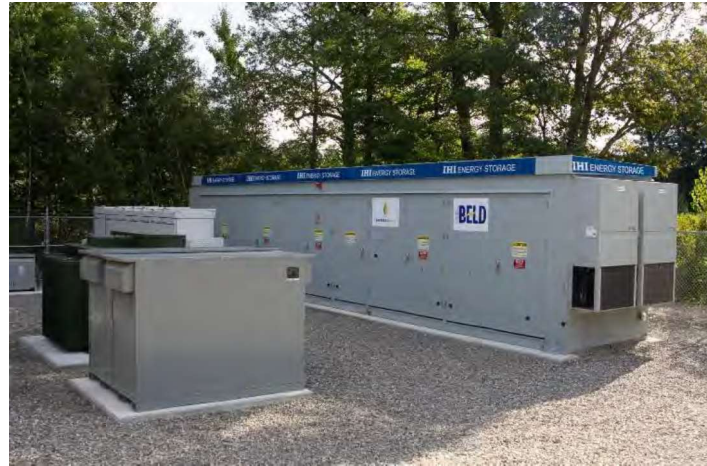
Example of an energy storage battery enclosure (right of picture) and inverter / transformer (left of picture)
