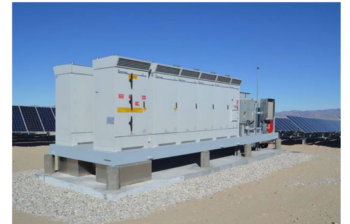
Inverter/Transformer Skid
