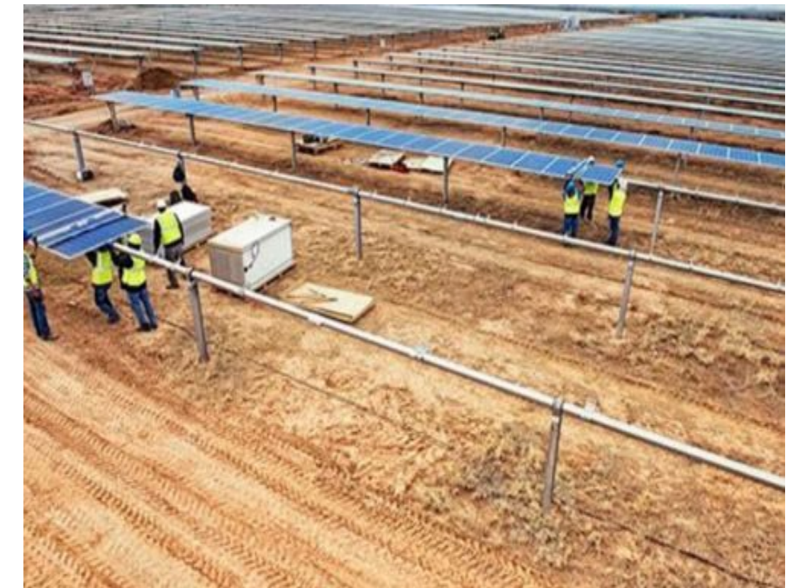
Panels installed on racking
