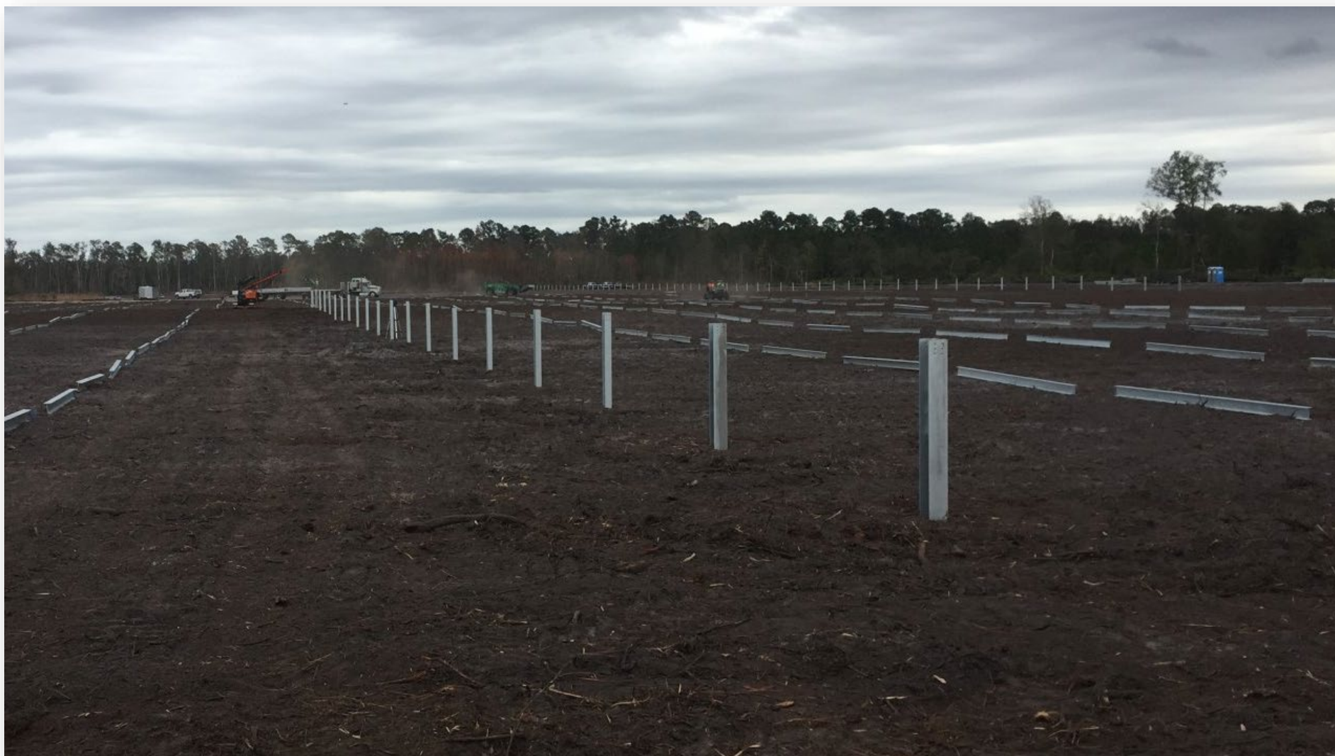
Driven pile foundations being installed at EDFR's project in Jacksonville FL
