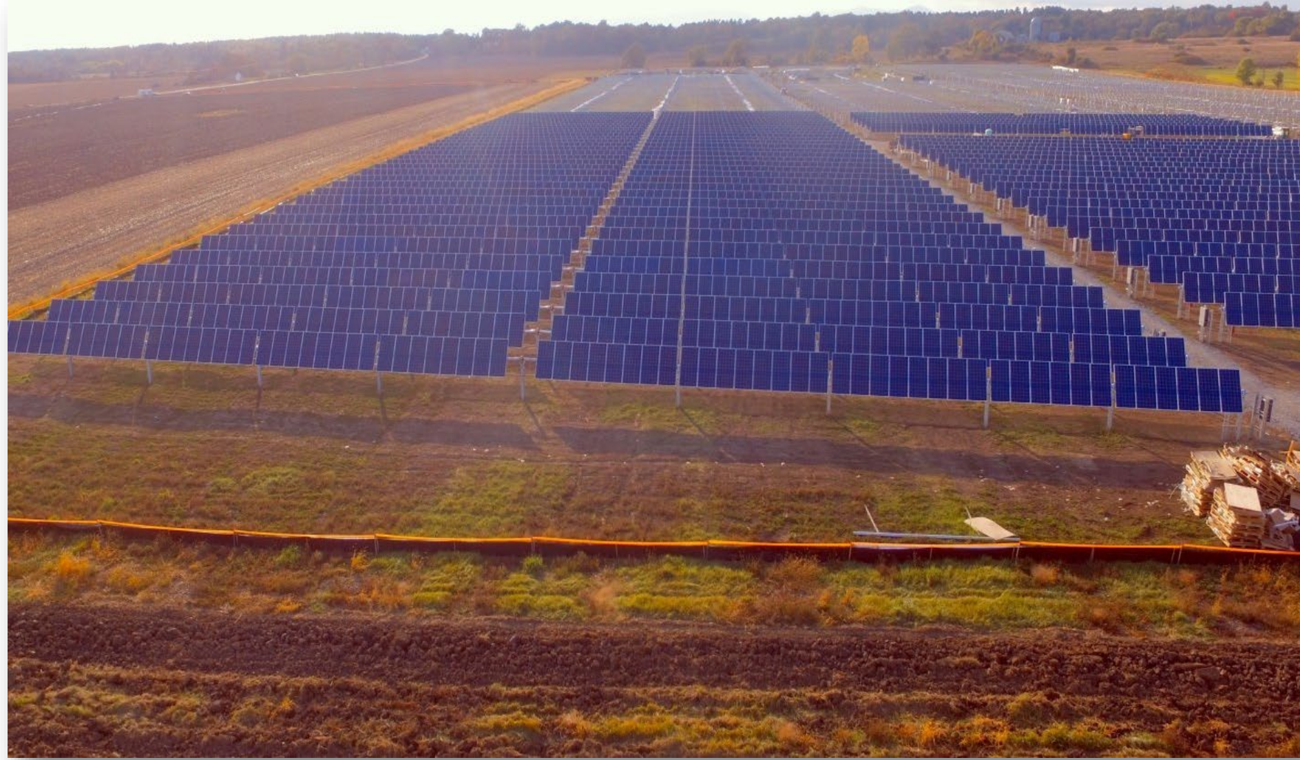
EDFR's Panton Project in Construction in Vermont
