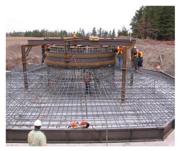
Figure 4-1: Preparation of a Typical Concrete Tower Foundation
