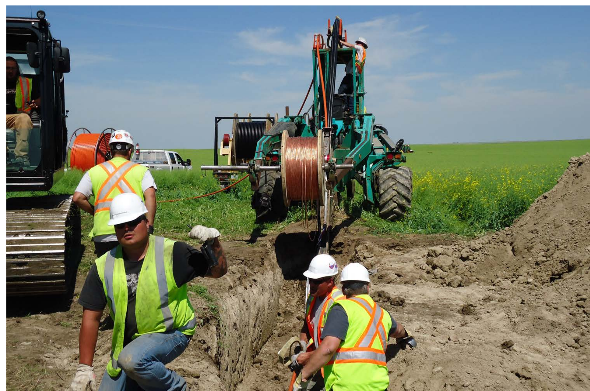
Buried collection system
