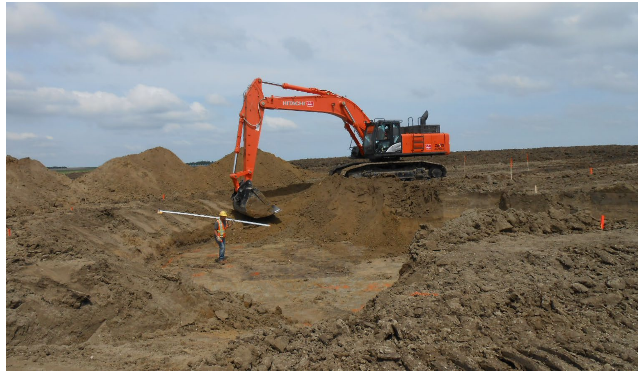
Foundation excavation. Diameter approx. 20 metres (m)
