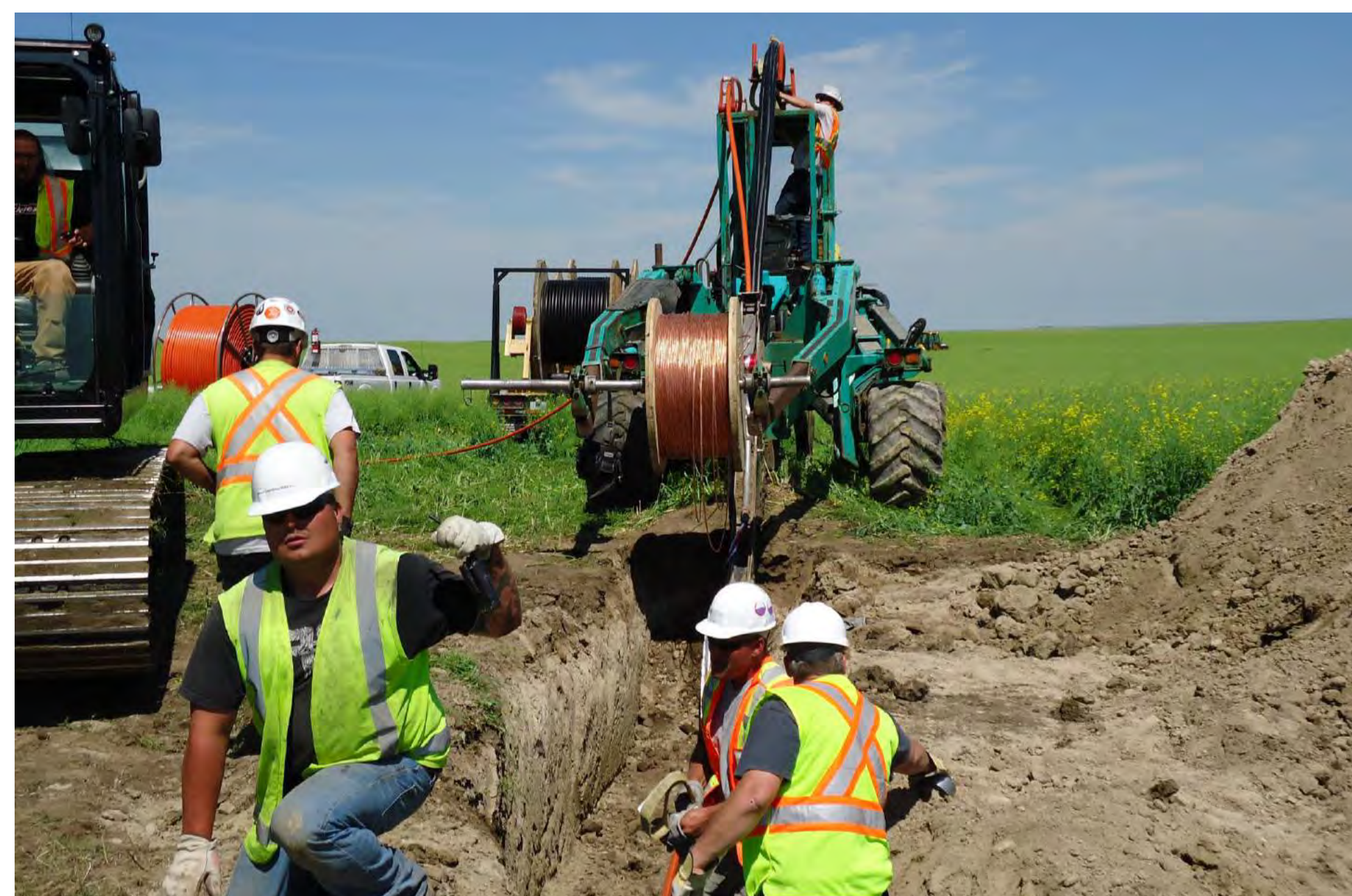
Buried collection system
