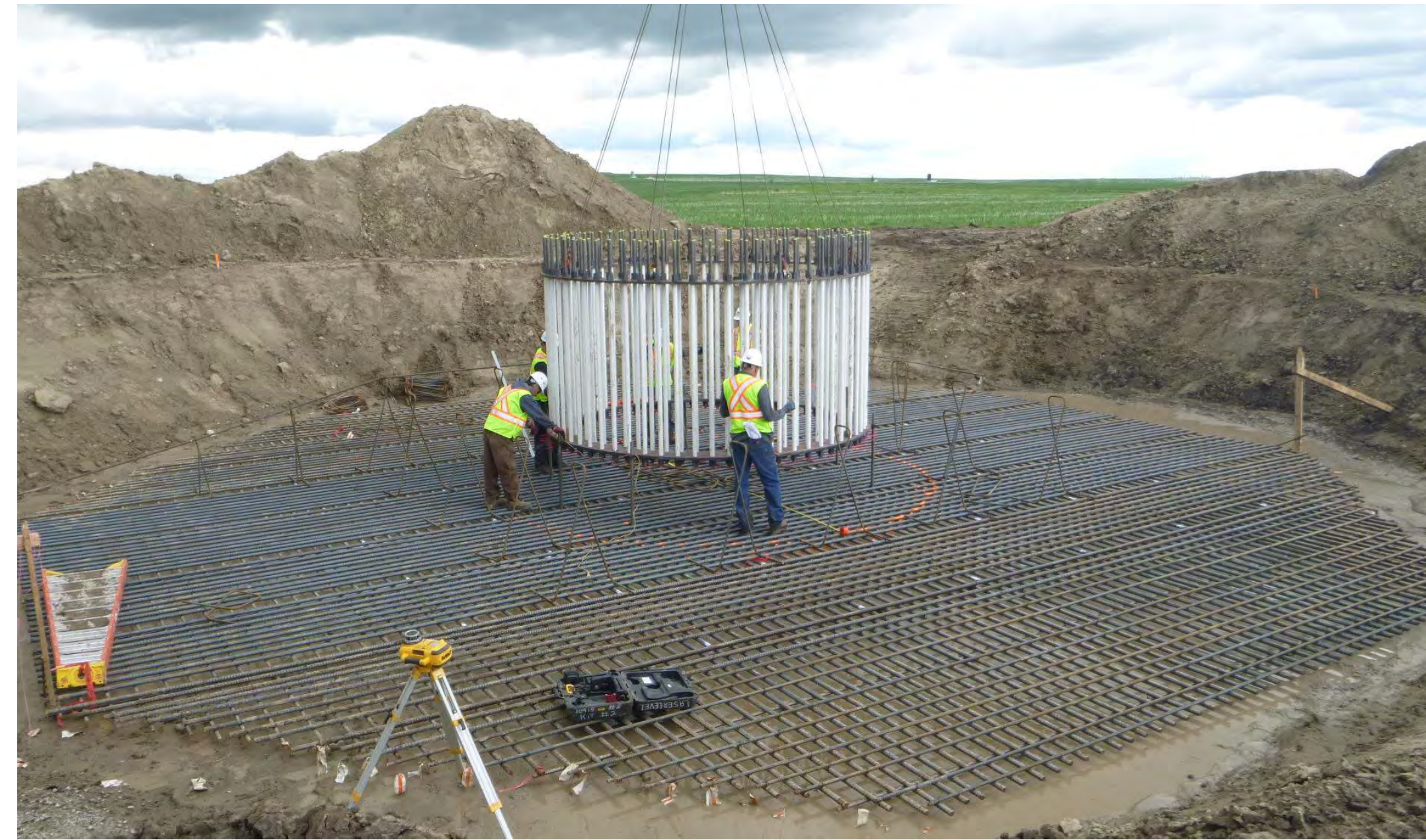
Reinforcing steel installation. Between 40-50 tons of rebar
