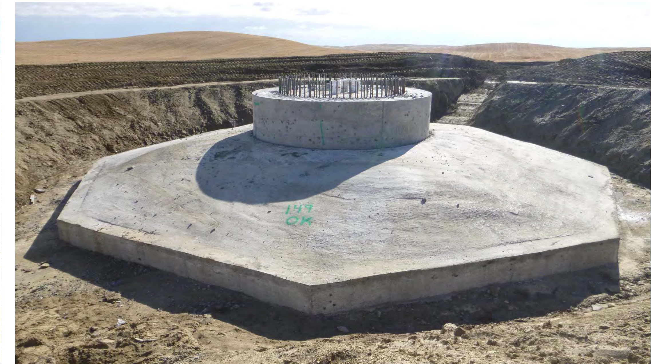
Each foundation requires approx. 400-600 m 3 of concrete.
