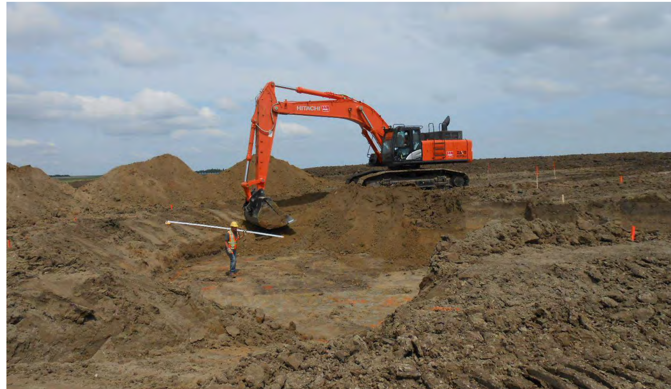
Foundation excavation. Diameter approx. 20 m
