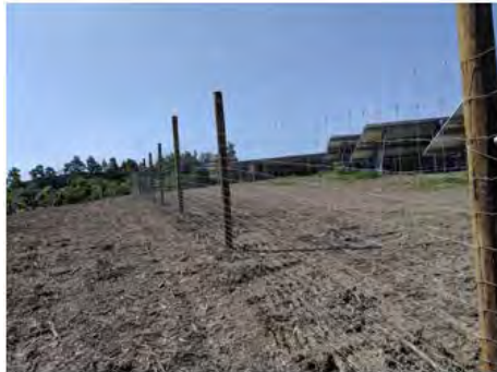
Agricultural Style Wire Knot Fence (Array Areas)
