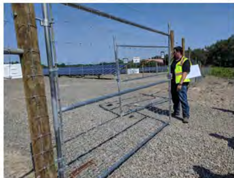
Typical Access Gate for Array Areas
