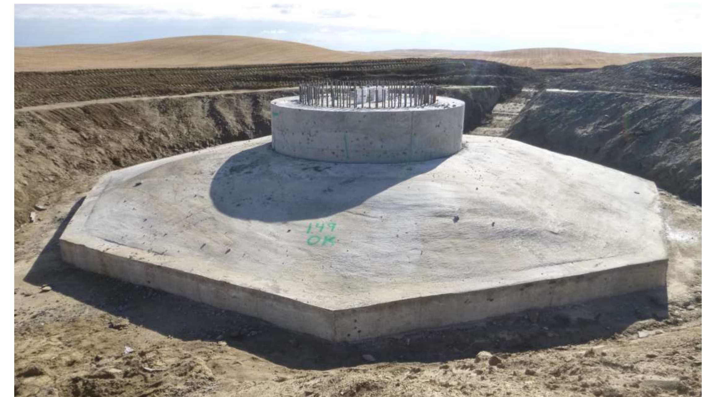
Each foundation requires approx. 400-600 m 3 of concrete.
