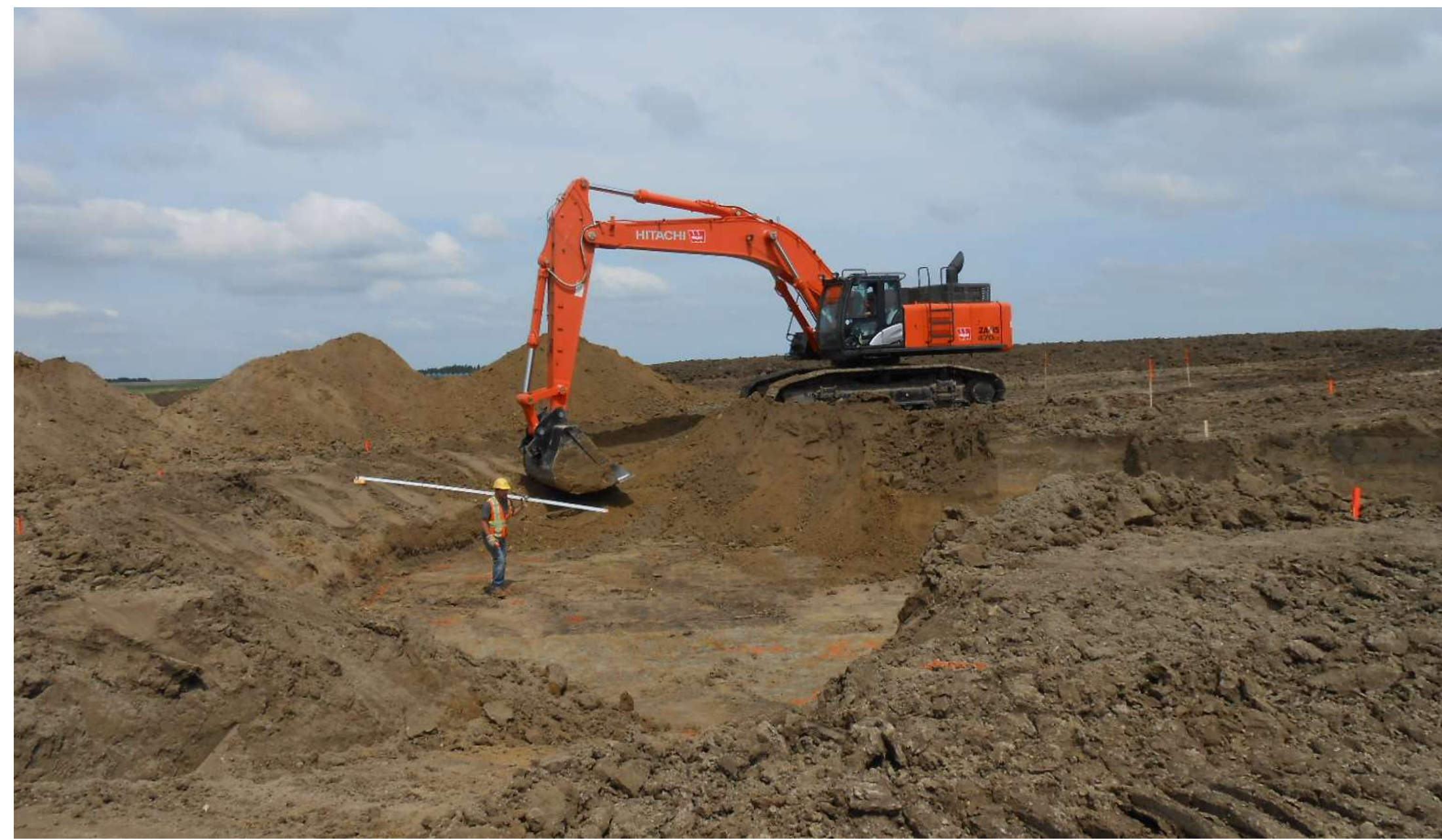
Foundation excavation. Diameter approx. 20 m
