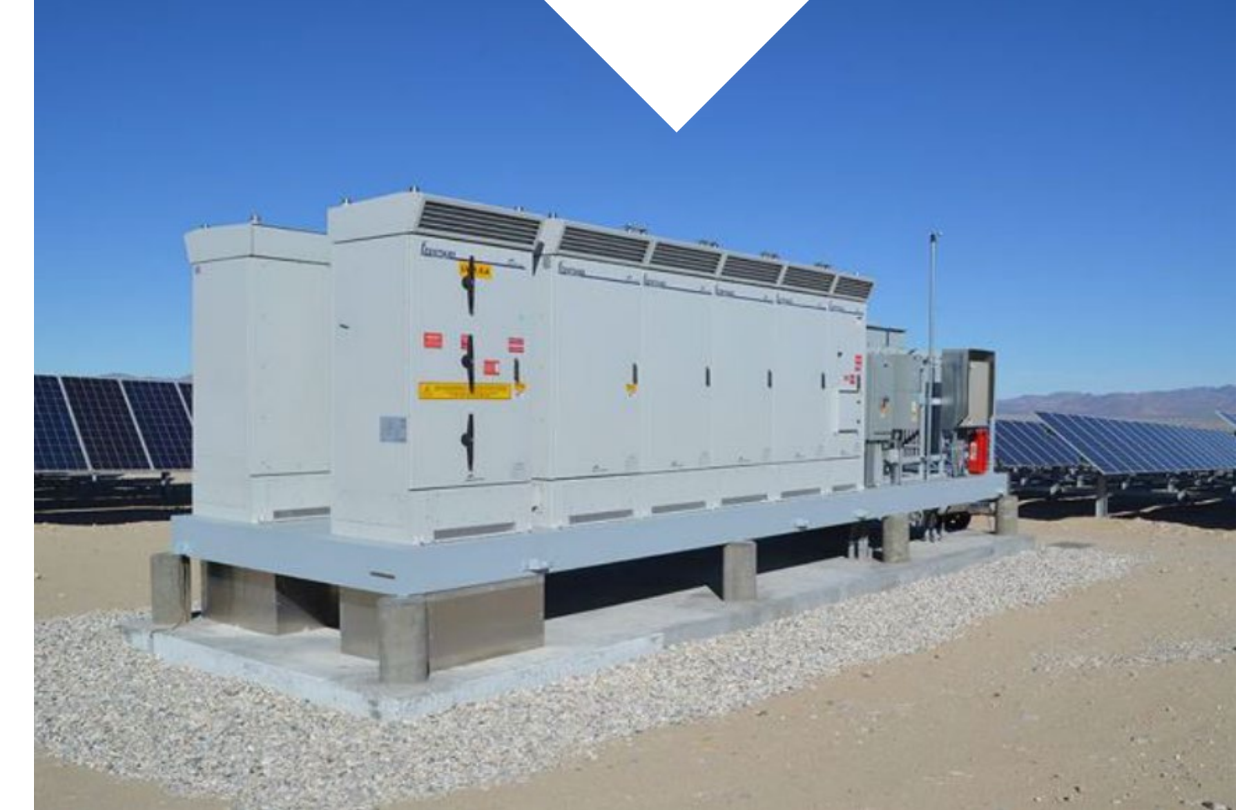
Inverter/Transformer Skid
