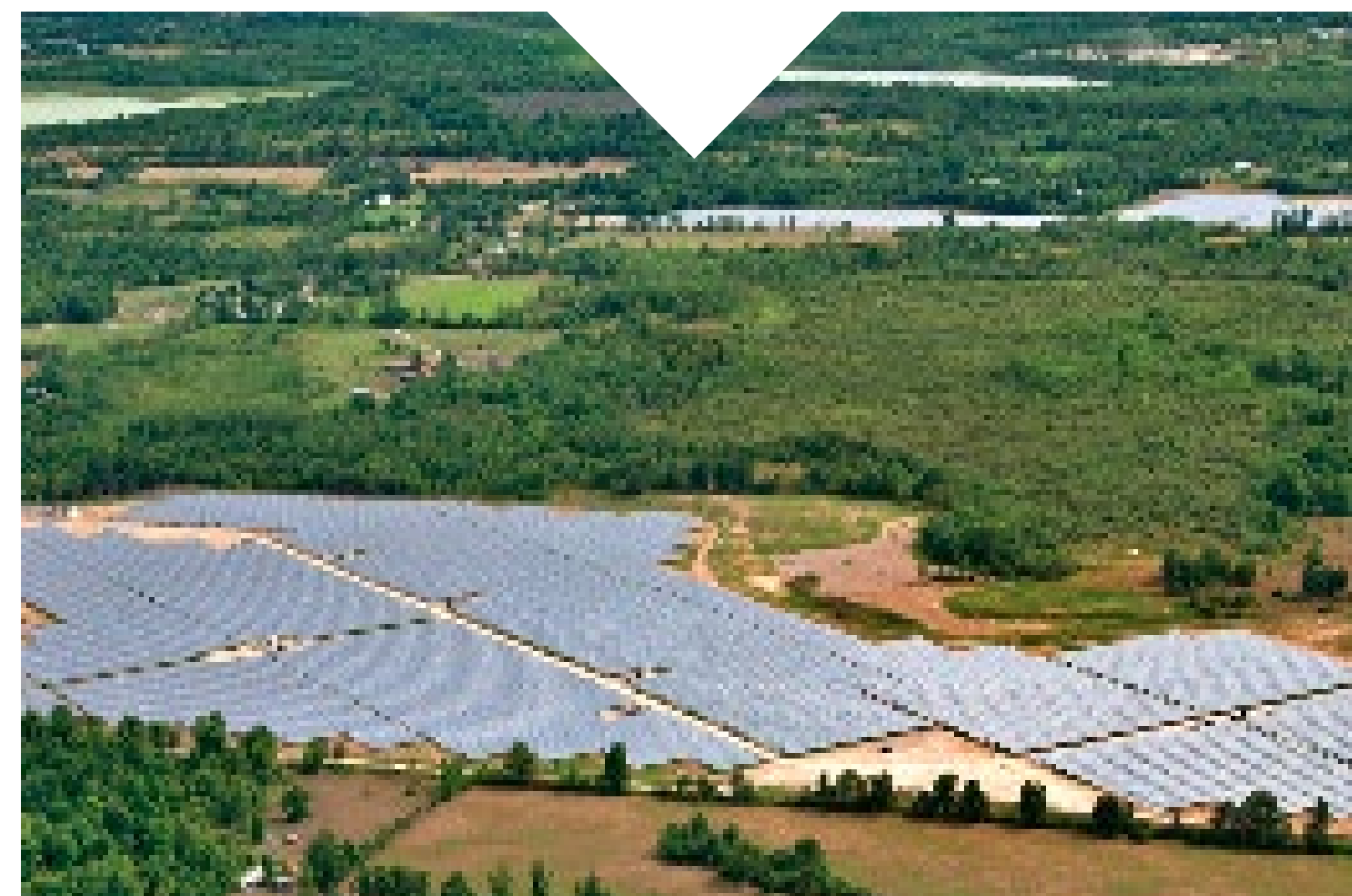
Aerial view of project
