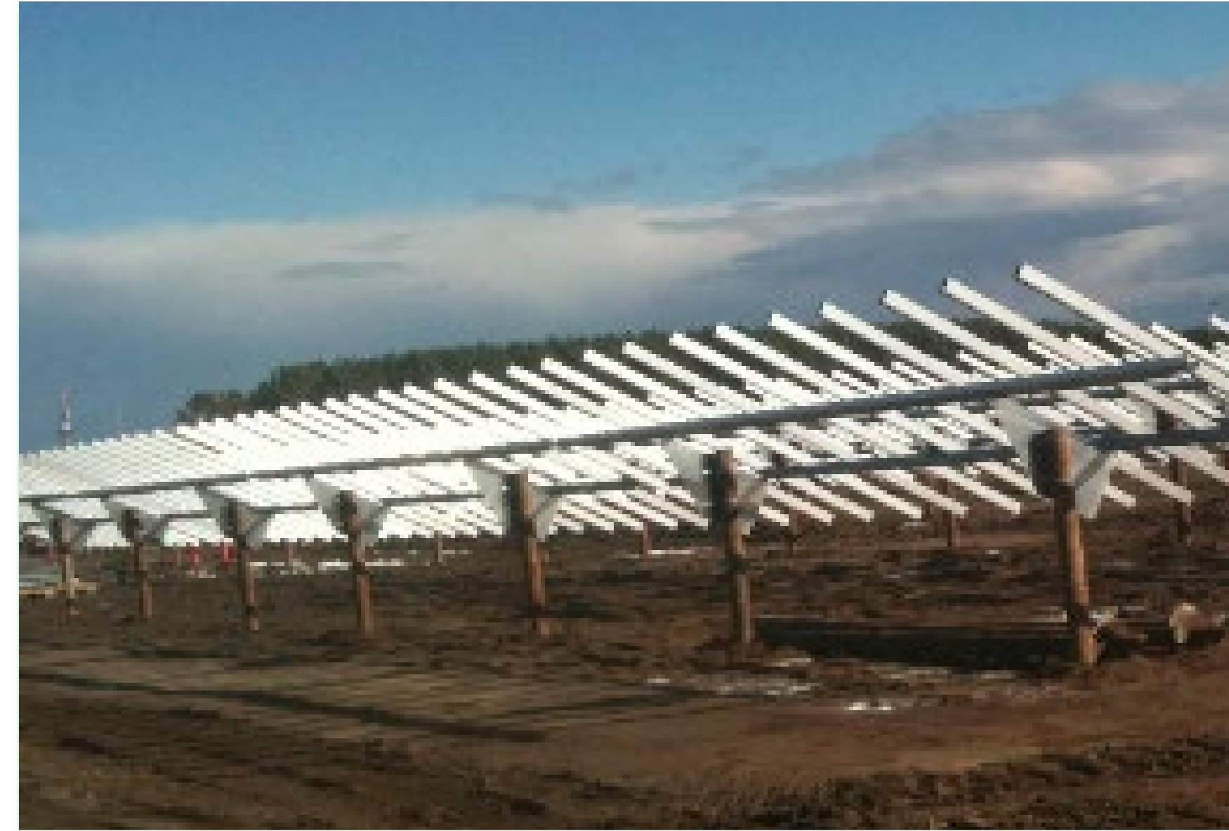
Racking mounted on piles
