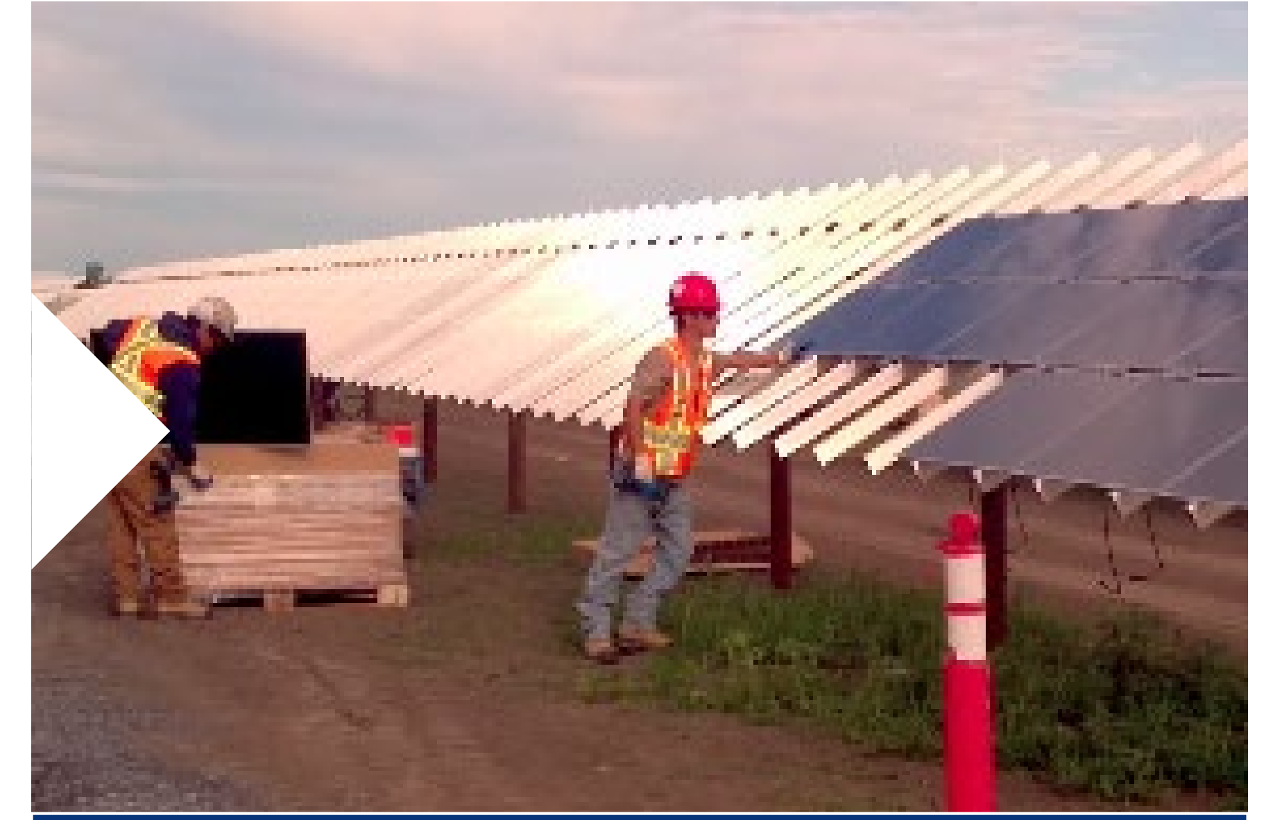
Panels installed on racking
