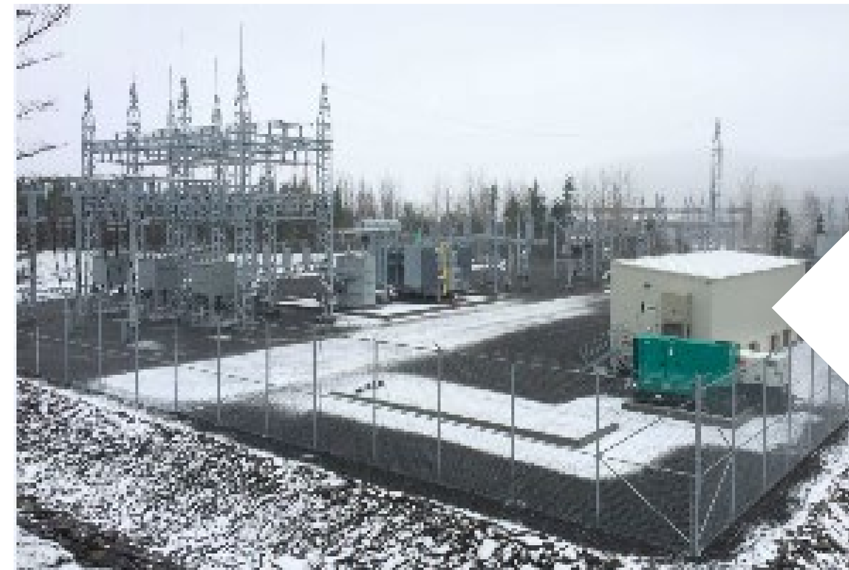
Project substation (grid tie)
